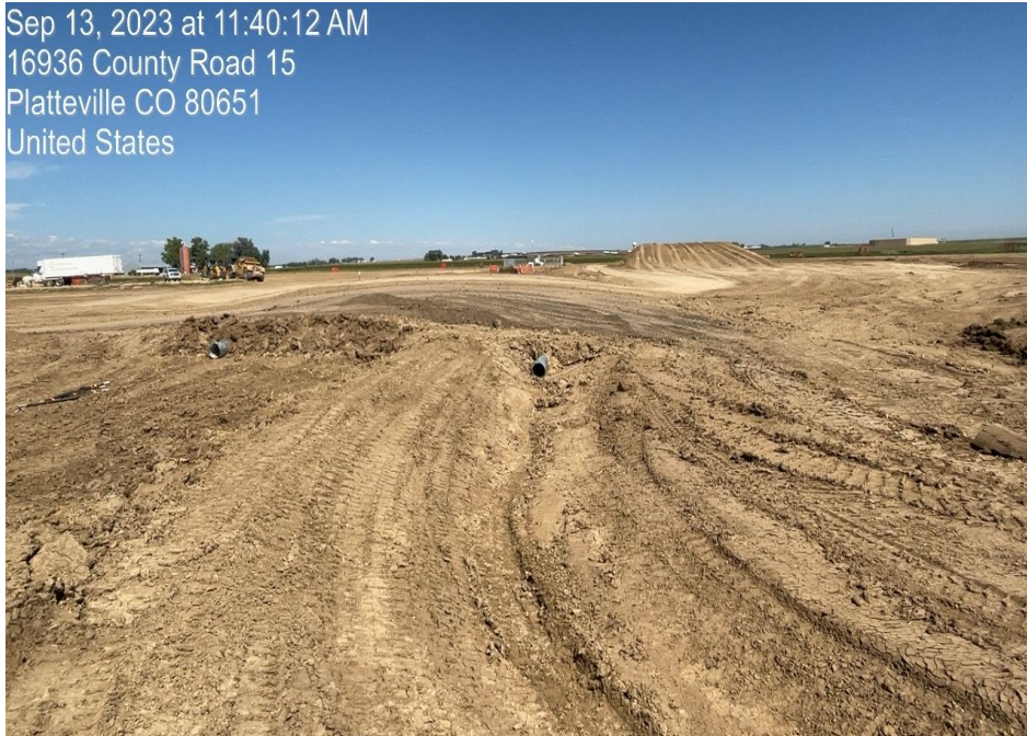
Photo 9. Photo taken of pipeline right of way crossing the location (construction is prohibited on the pipeline). Photo taken facing north, of culverted vehicle crossing point across pipeline right of way.
