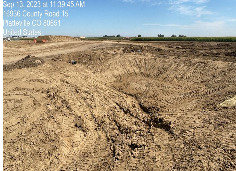
Photo 10. Photo taken of large sediment trap on southeast corner of site. Photo taken facing north. (site under construction)
