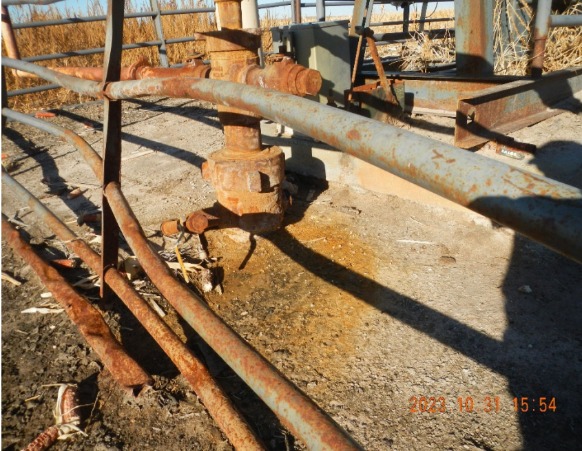
3. Additional view of staining around wellhead and damaged stock panels.
