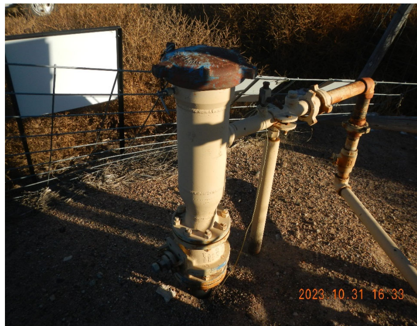
10. Pig station at remote gas meter location.
