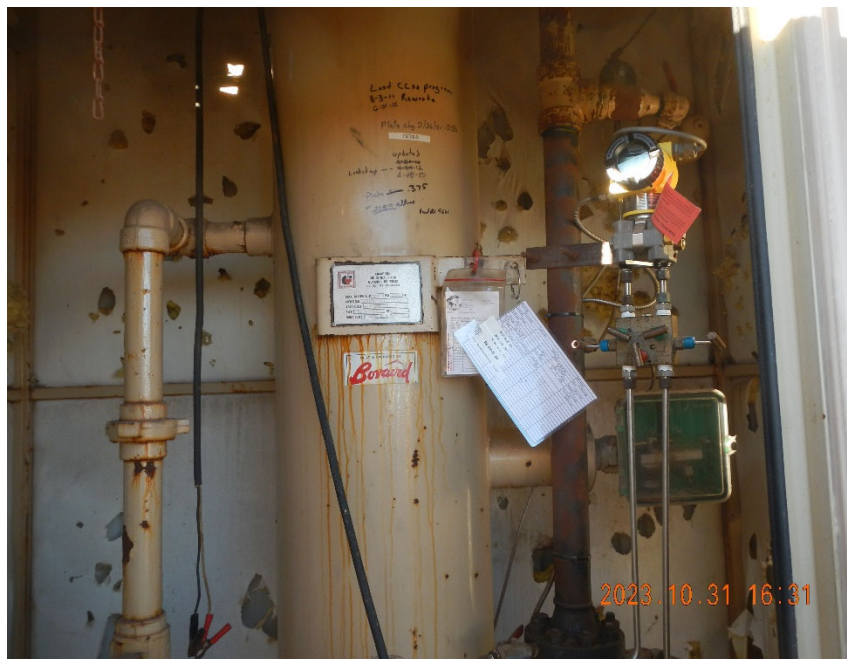
9. Vertical separator and digital gas meter inside shed.
