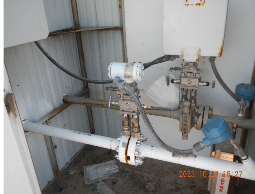
6. Digital gas meter. Calibration log needs to be replaced.
