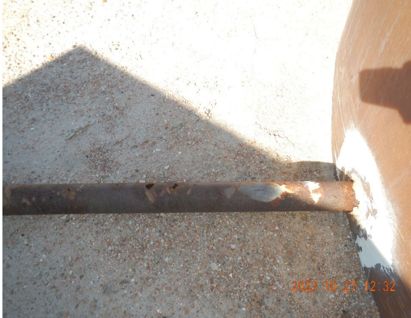
7. Holes in dump line prior to tank tie in.
