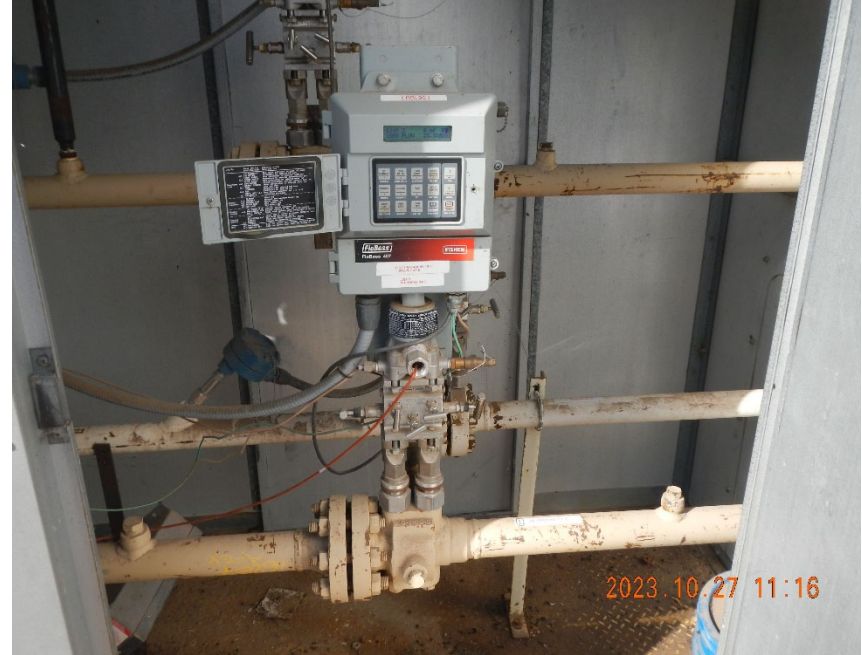
6. Digital gas meter run.
