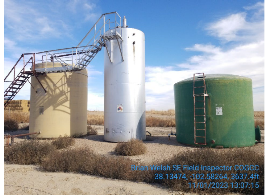
West side of tanks looking east
