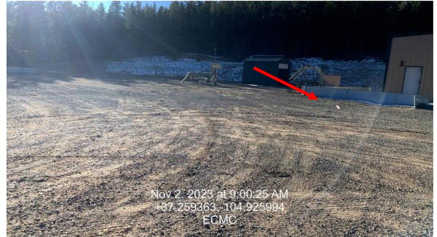
**Photo 5 – Oil Stained Gravel in Secondary Containment**
