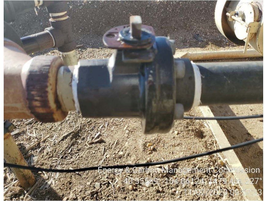
Valve leak
