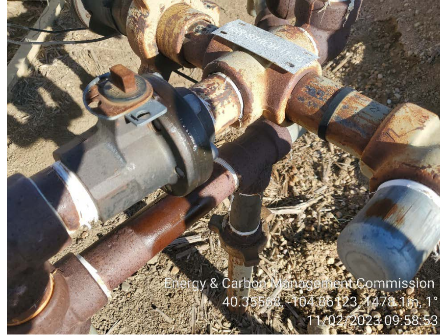
Valve leak
