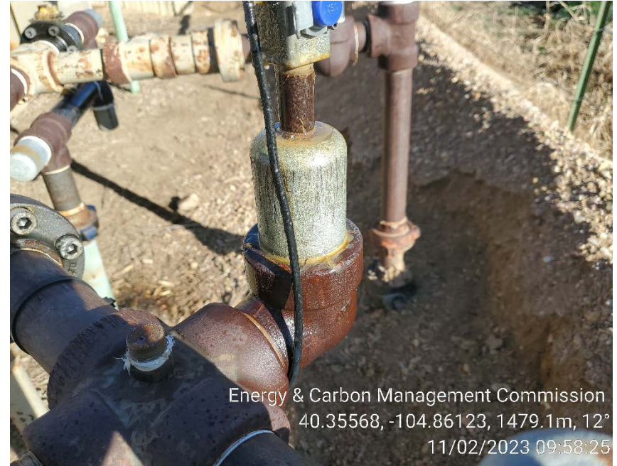
Valve leak
