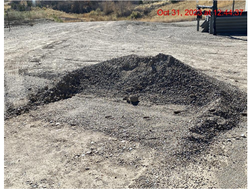
Unprotected Soil Stockpile – Photo #07275
