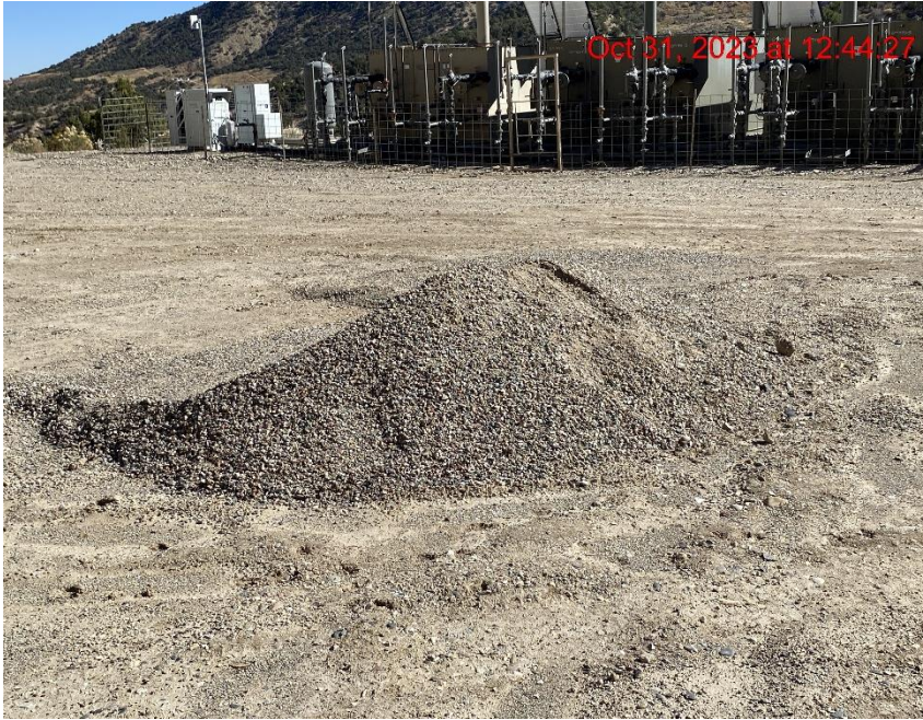
Unprotected Soil Stockpile – Photo #07274
