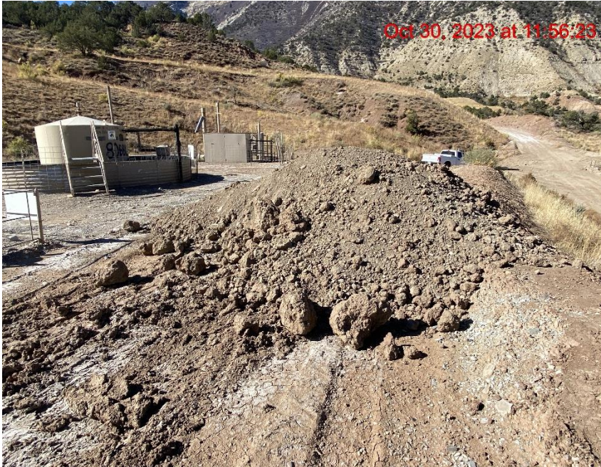
Unprotected Soil Stockpile – Photo #07243
