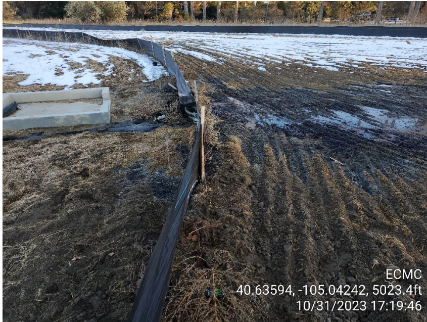
Photo 3: Looking at inlet to rain garden with oil/produced water visible impacts
