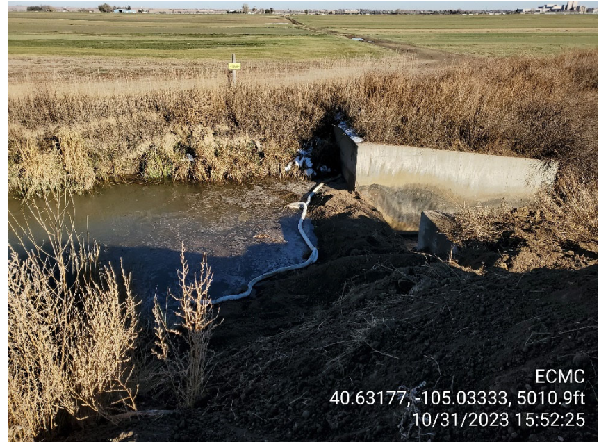
Photo 18: View of temporary berm constructed downstream in Number 8 Outlet ditch.
