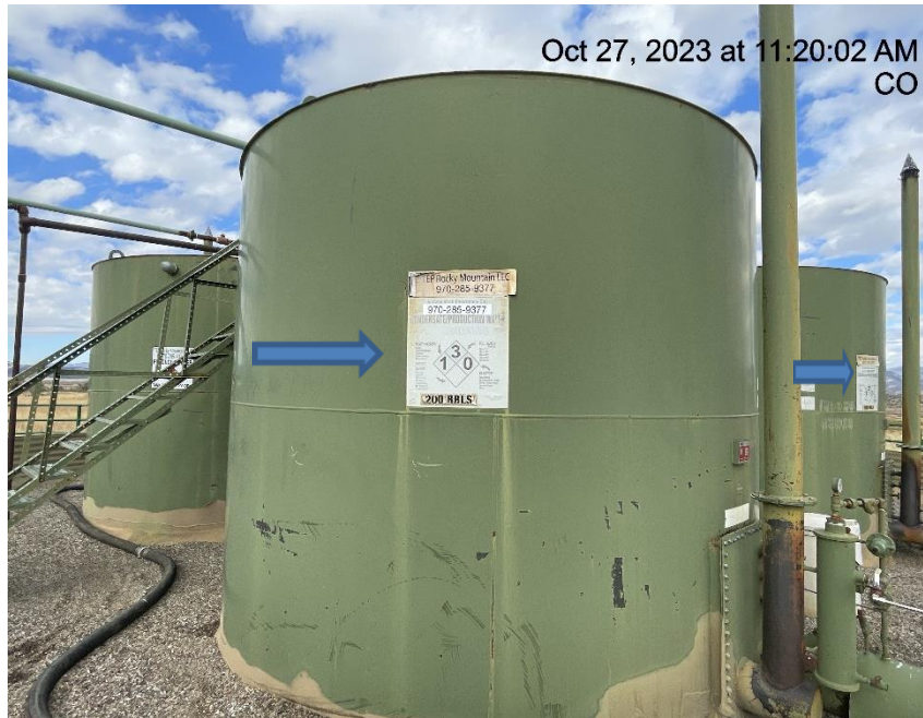
Photo # 4517 Multiple tank labels are weathered & fading
