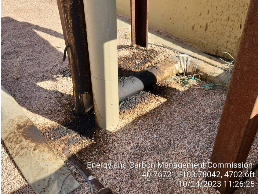
Photo 5 – Stained Soil at Recycle Pump
