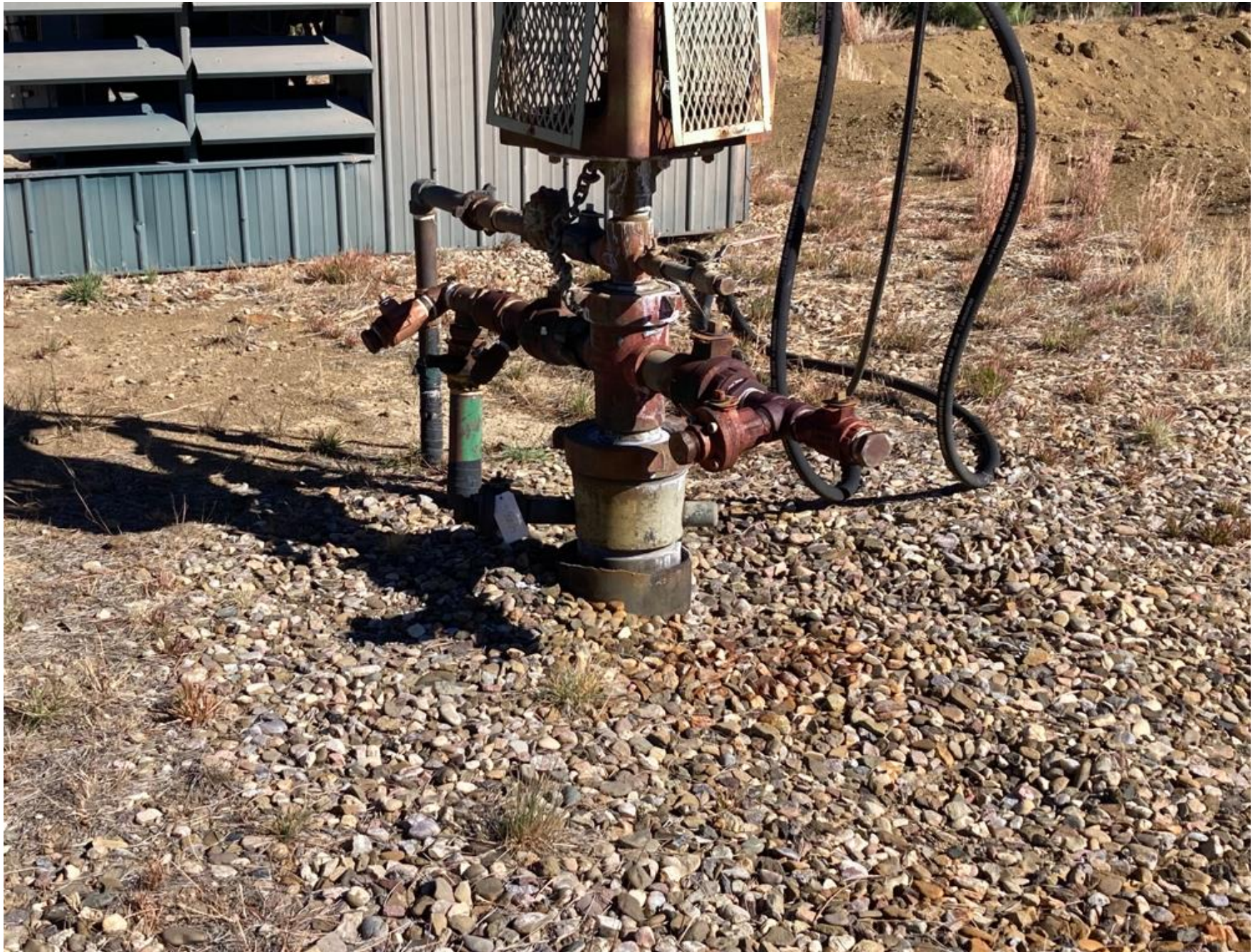
PHOTO 1: THE CONTAMINATED SOIL HAS BEEN REMOVED FROM LOCATION. EQUIPMENT MAINTENANCE HAS BEEN PERFORMED AND THE SELF INSPECTION PROCESS REVIEWED.
