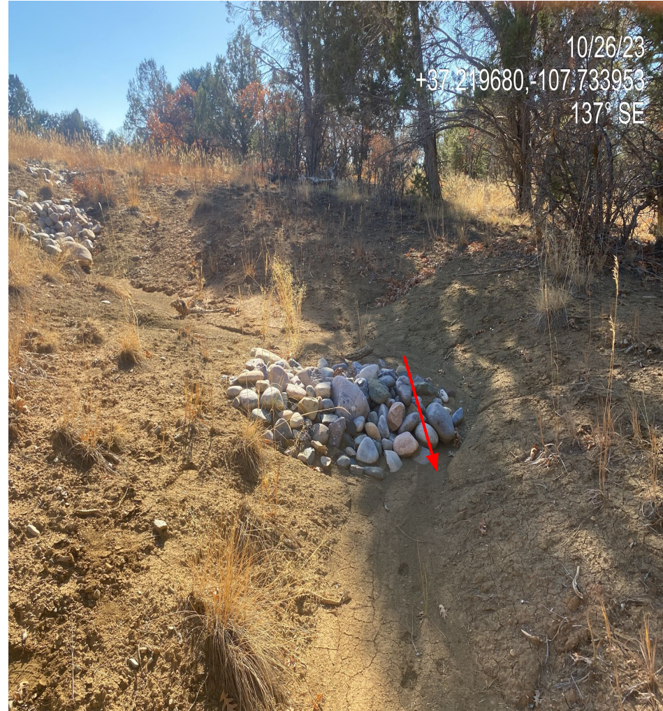
Photo 4. View of stormwater BMPs in the southern interim reclamation area. Erosional scouring and sediment transport remains.
