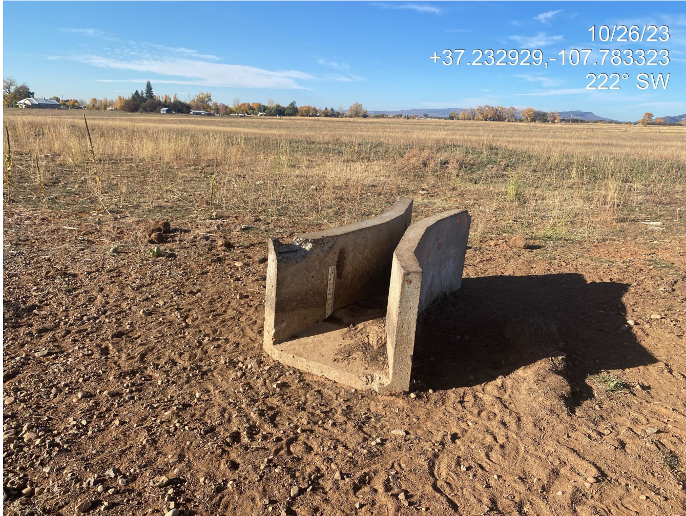
Photo 3. Debris observed on the western edge of the disturbance.
