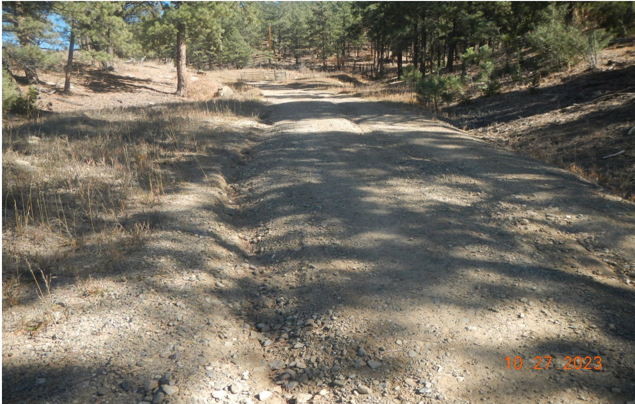
Photo 1. Facing northwest toward the access road. There is erosion along the road that needs to be repaired..
