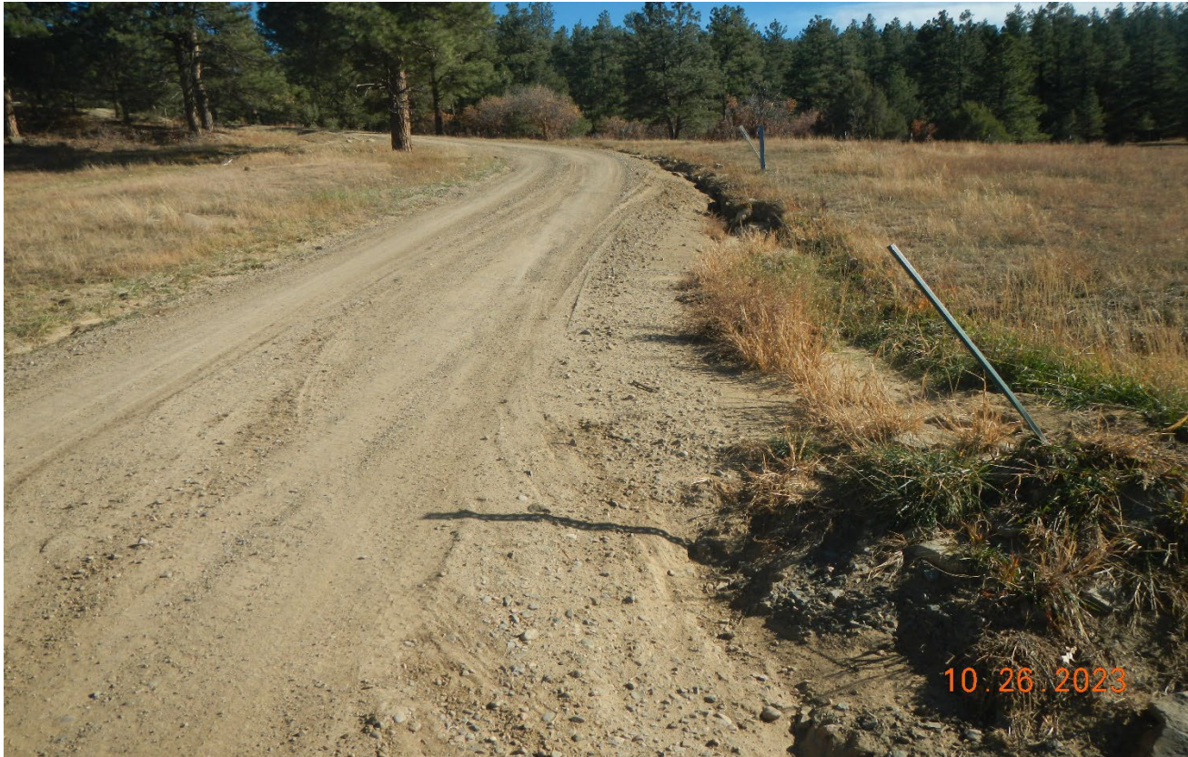
Photo 1. This culvert along the main access road is filled in with sediment at Lat/Long:37.302109, -104.78223 .
