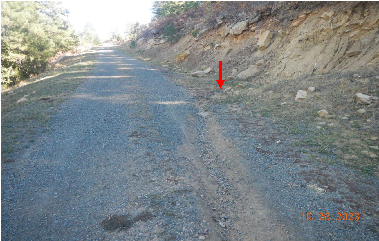
Photo 5. Facing southeast along the access road. The culvert at the red arrow is filled in with sediment and which is causing stormwater to flow down the road.
