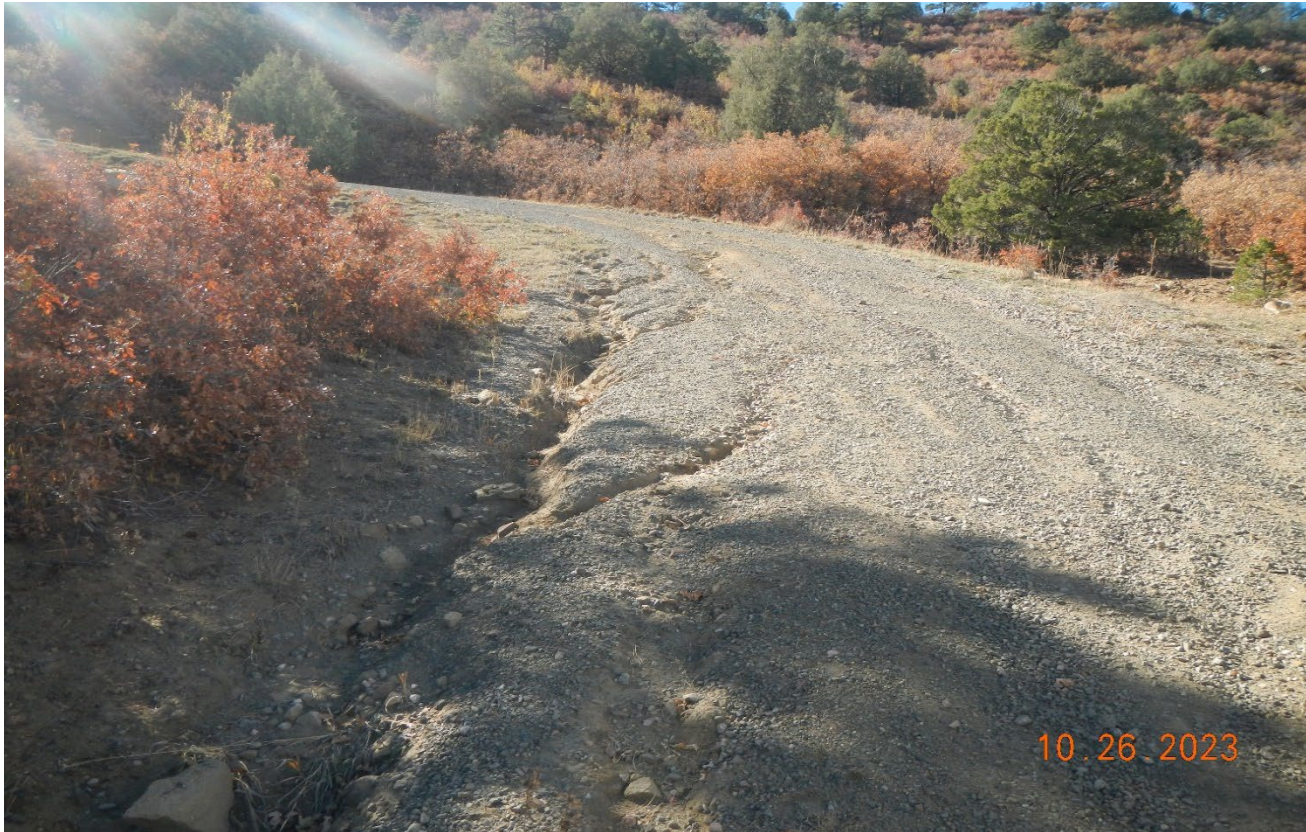
Photo 3. Facing southwest along the switch back of the access road which has erosion issues.
