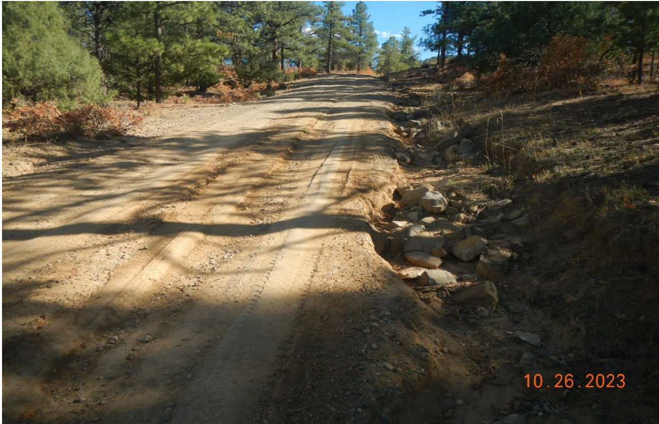
Photo 2. There is erosion along the roadside near the Rampart 43-33 well site.
