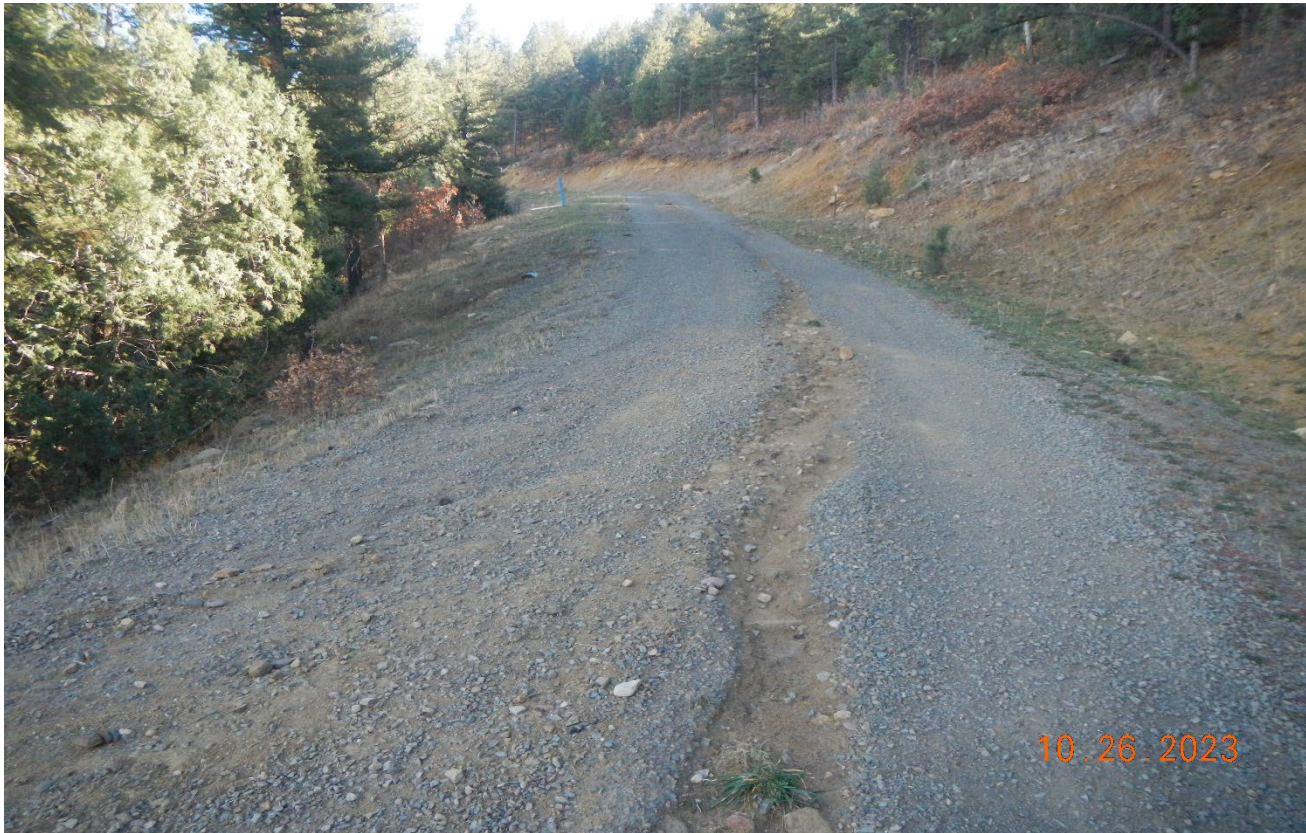
Photo 4. Facing southeast along the access road. There is erosion occurring down the center of the road.
