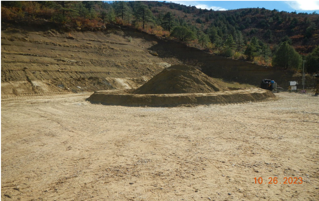
Photo 1. Facing southeast at the location. There is a pile material that remains at the location with a compacted berm.
