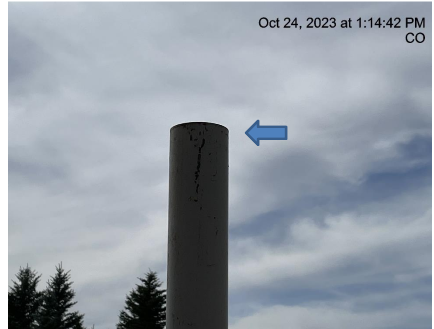
Photo # 4095 Open ended pipe on production tank/wildlife hazard
