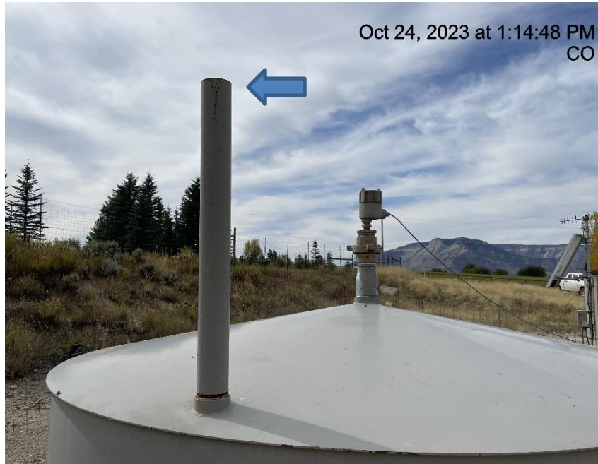
Photo # 4094 Open ended pipe on production tank/wildlife hazard
