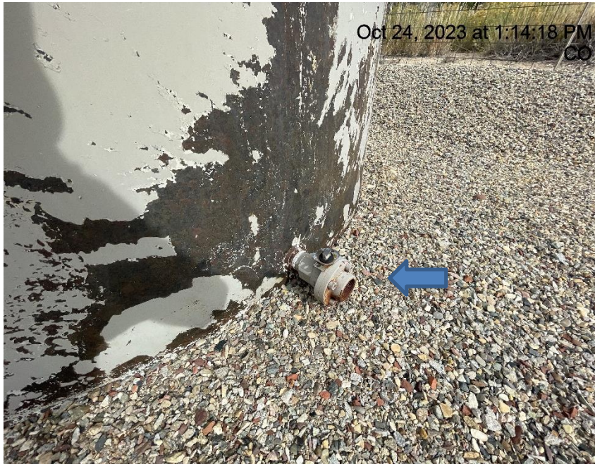
Photo # 4096 Open ended load line
