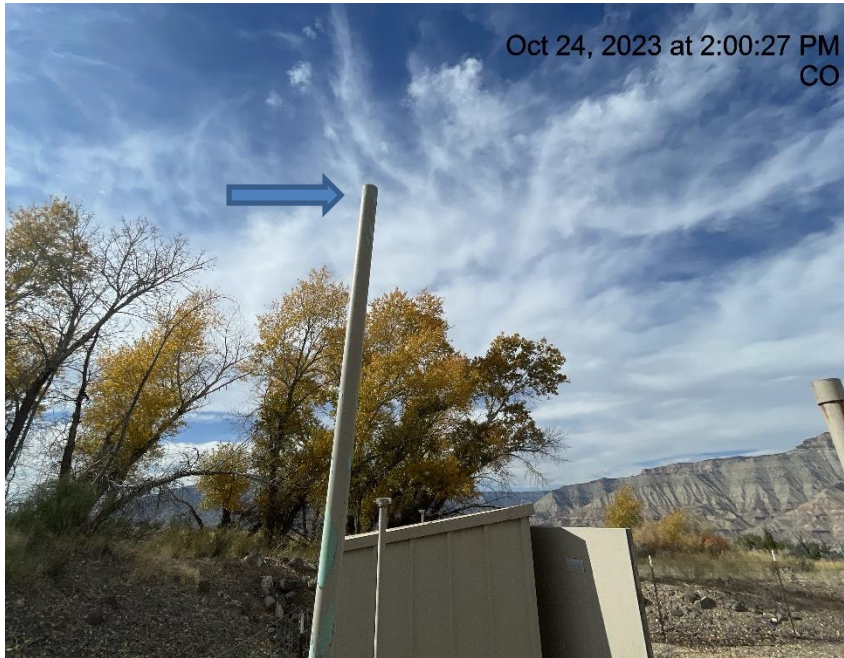
Photo # 4177 Open ended pipe/wildlife hazard
