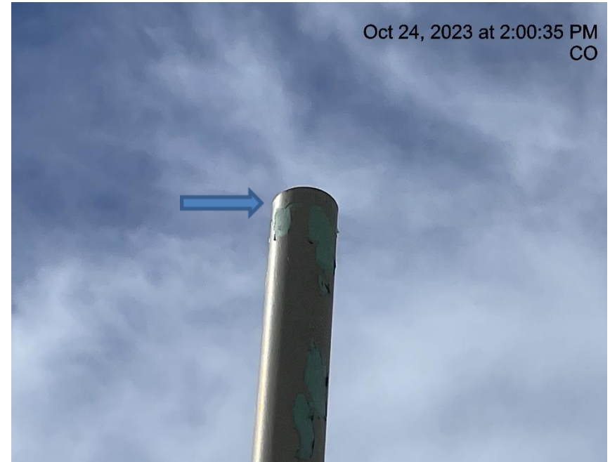
Photo # 4178 Open ended pipe/wildlife hazard
