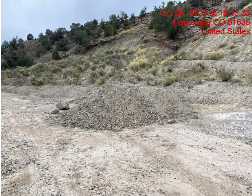
Unprotected Soil Stockpile – Photo #07178
