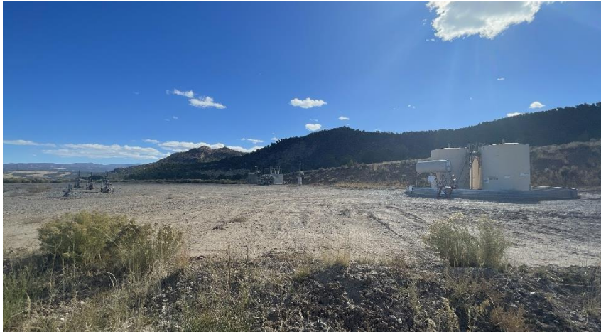
North West corner of location.
