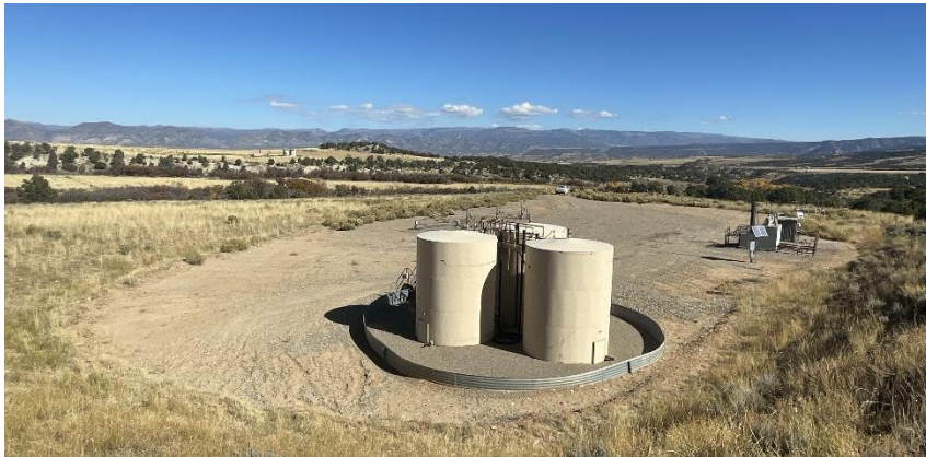
South West corner of location.
