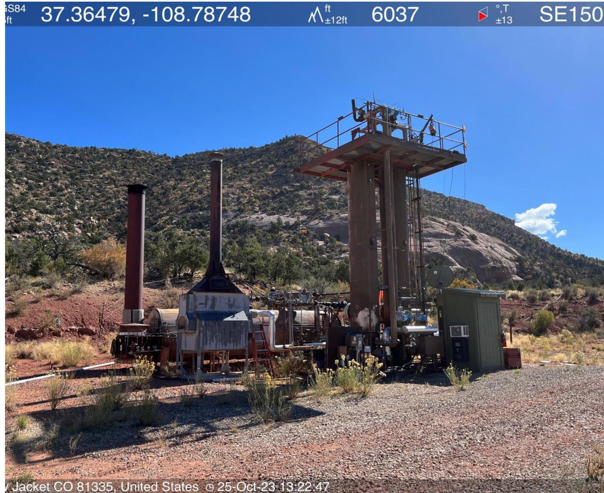
**Photo #8 View of heated separators and vertical gas scrubbers.**
