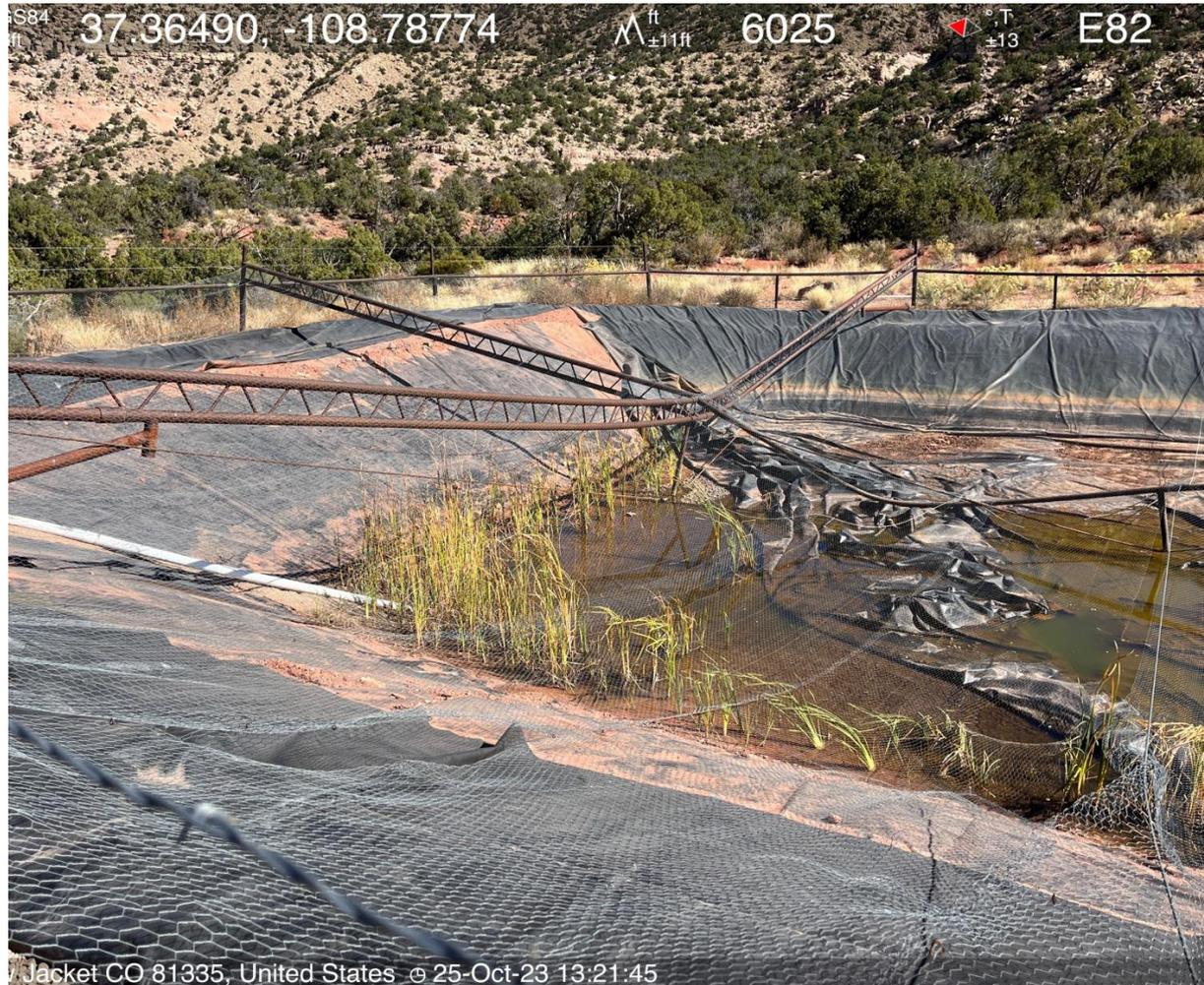
Photo #6 View of pit liner and netting supports.
