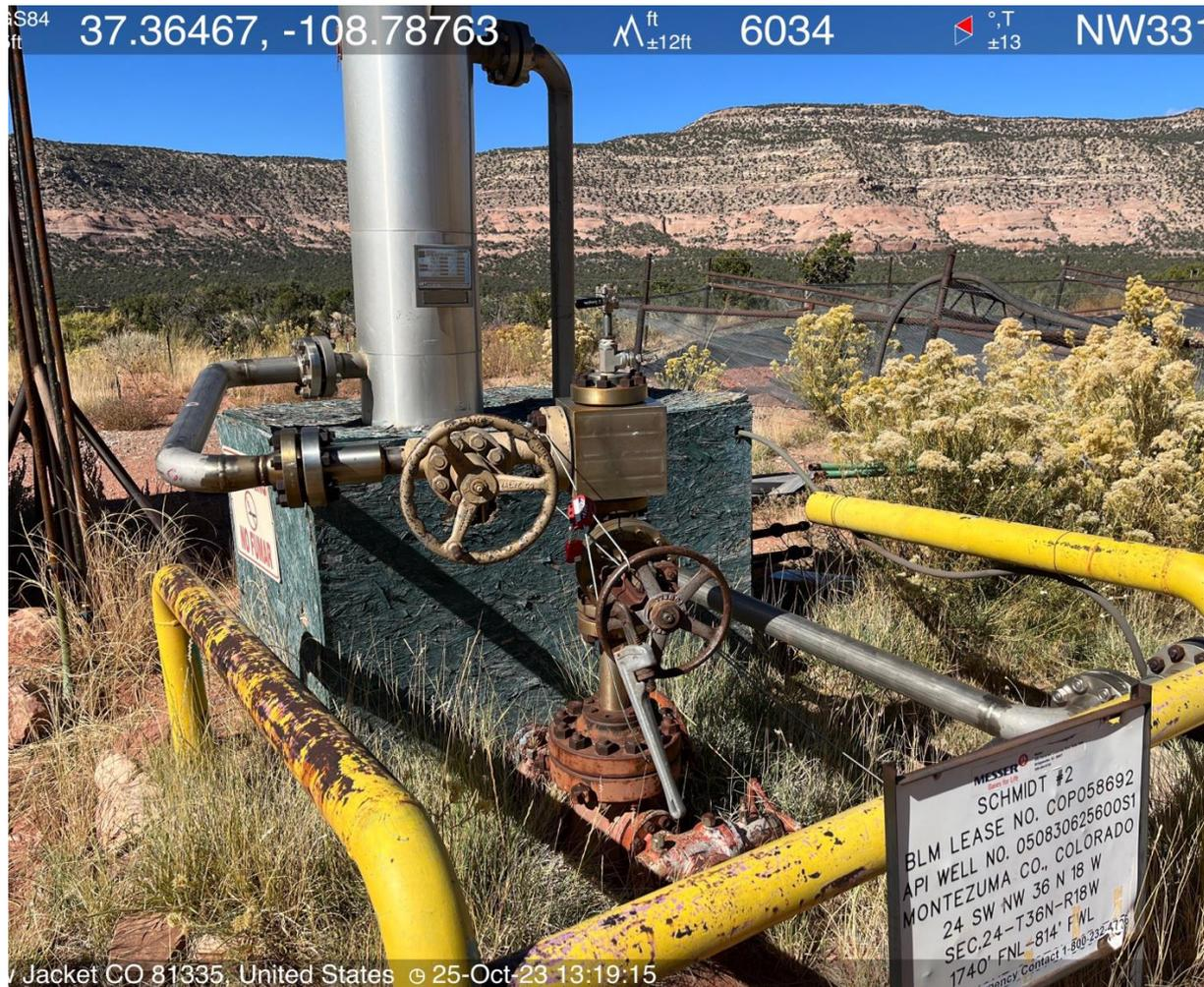
Photo #4 View of the wellhead assembly.
