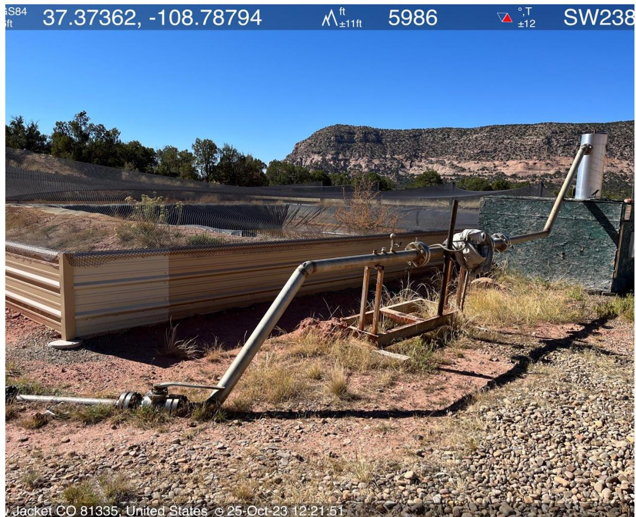
Photo #7 View of meter run and surface gathering line.
