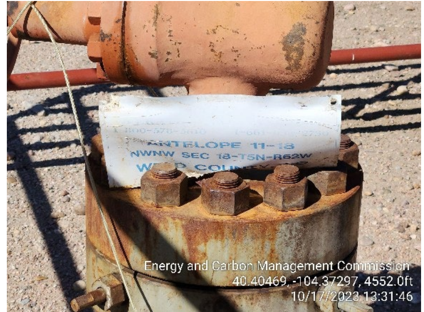
Photo 2 – Wellhead Sign – 24 Hour Number no longer visible
