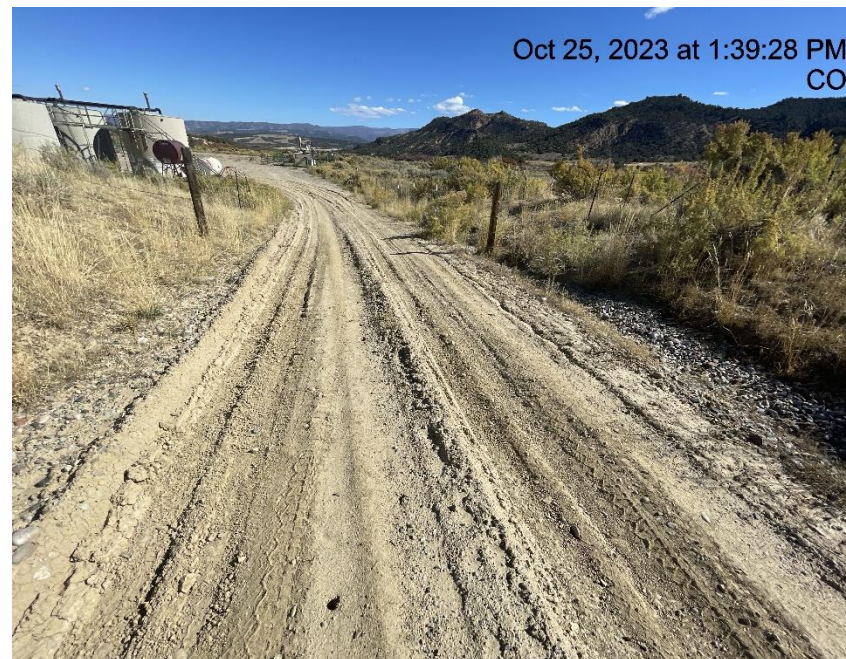
Photo # 4310 Lack of stabilization/compaction on lease road near entrance to location
