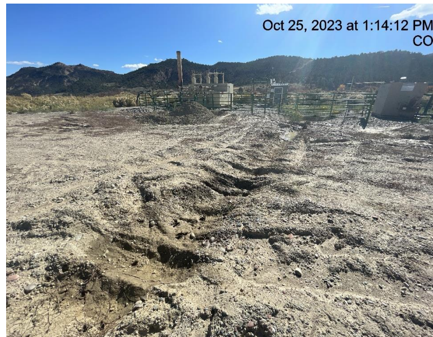
Photo # 4286 Lack of stabilization/compaction on location
