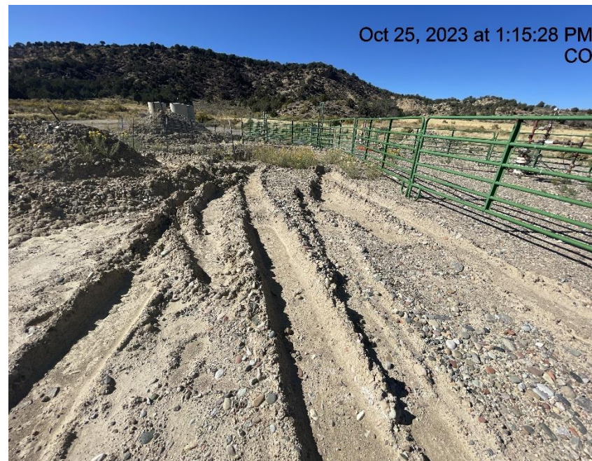
Photo # 4292 Lack of stabilization/compaction on location
