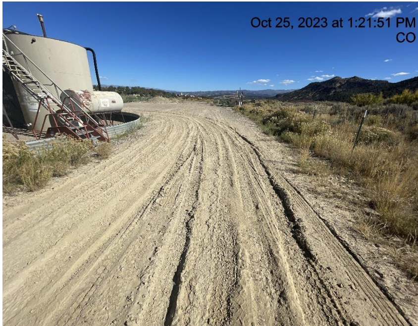
Photo # 4307 Lack of stabilization/compaction at entrance to location
