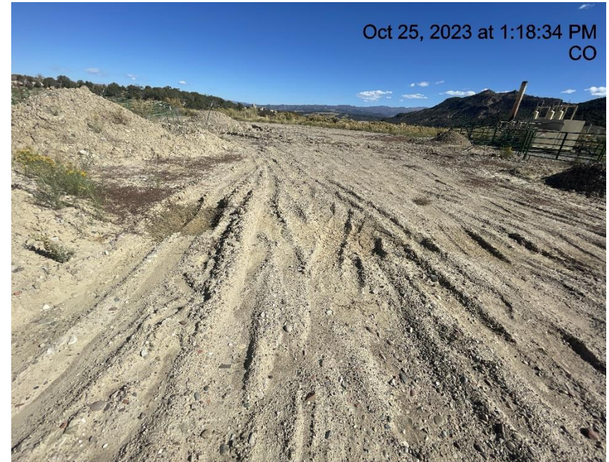
Photo # 4300 Lack of stabilization/compaction on location
