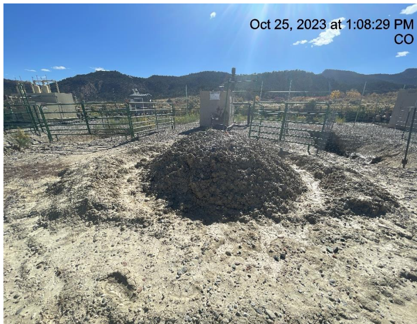
Photo # 4275 Berm around stockpiled soils has eroded/BMP needs maintenance
