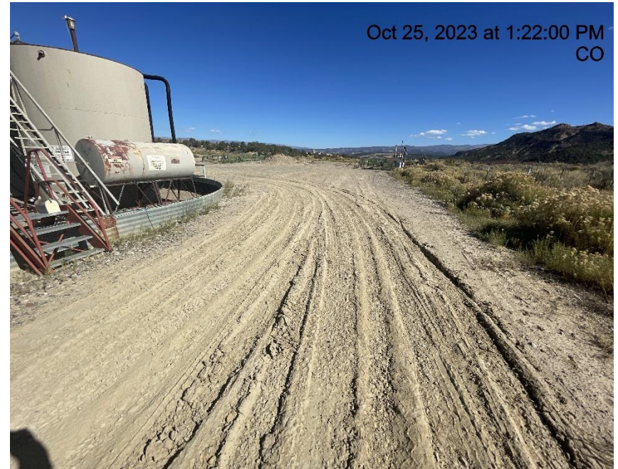
Photo # 4308 Lack of stabilization/compaction at entrance to location
