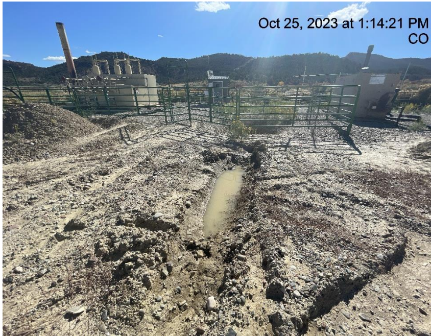
Photo # 4287 Lack of stabilization/compaction on location
