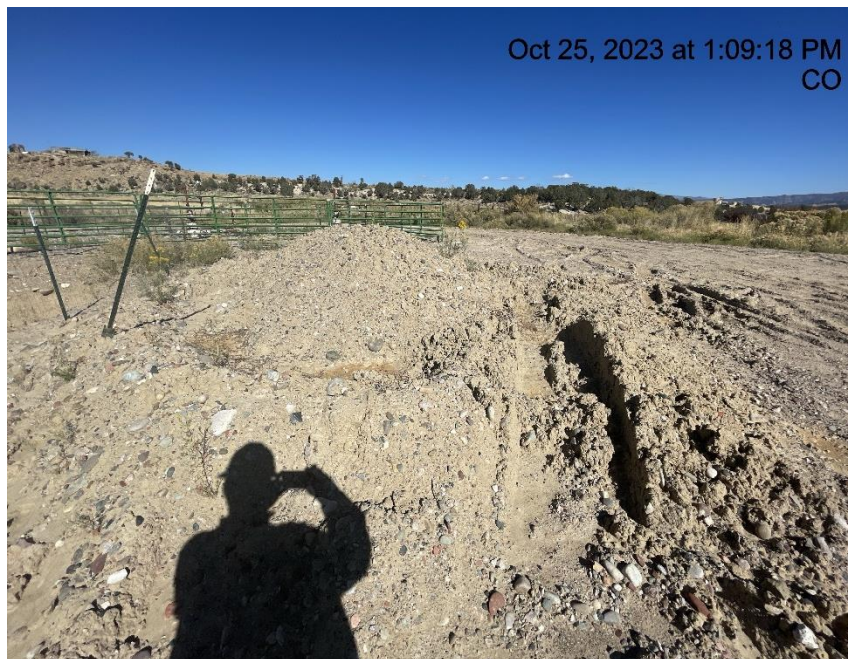
Photo # 4277 Vehicle tracks through berm around stockpiled soils/BMP needs maintenance
