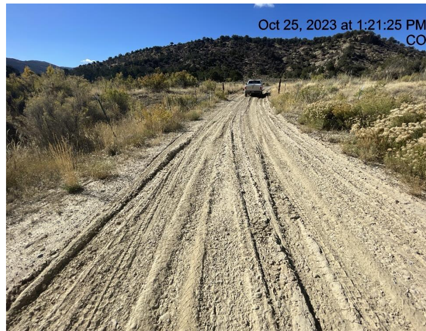
Photo # 4306 Lack of stabilization/compaction near entrance to location
