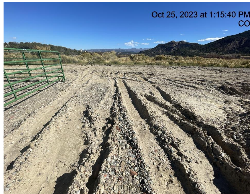
Photo # 4294 Lack of stabilization/compaction on location
