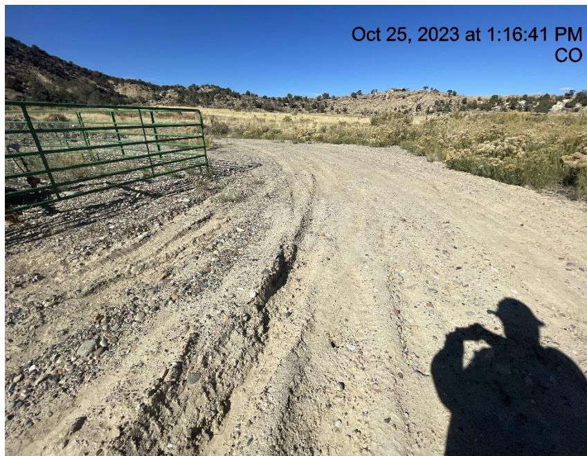
Photo # 4297 Lack of stabilization/compaction on location
