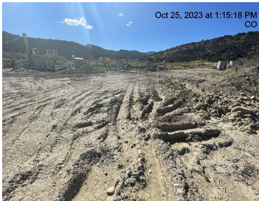
Photo # 4291 Lack of stabilization/compaction on location
