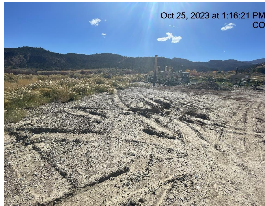
Photo # 4296 Lack of stabilization/compaction on location
