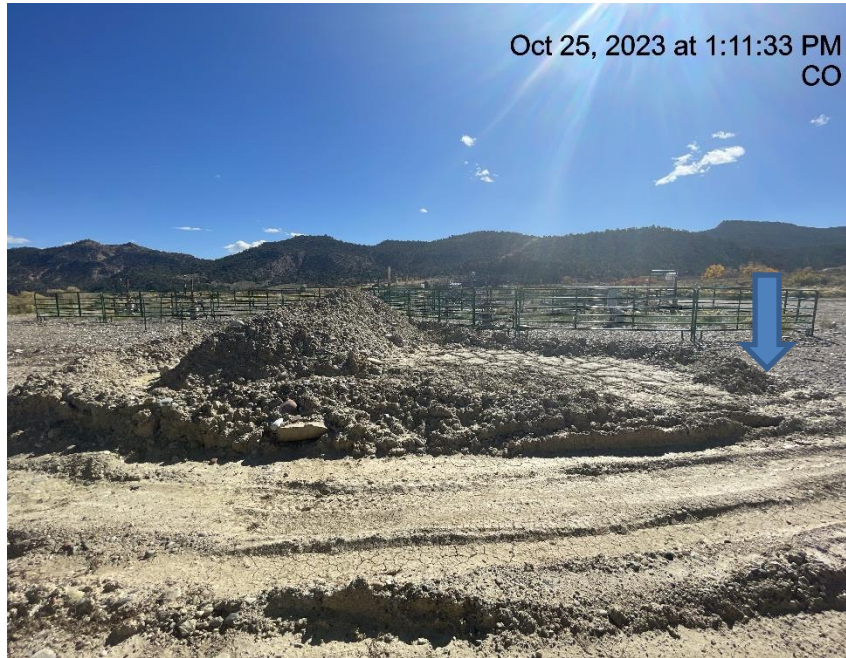
Photo # 4279 Berm around stockpiled soils has partially eroded/BMP needs maintenance
