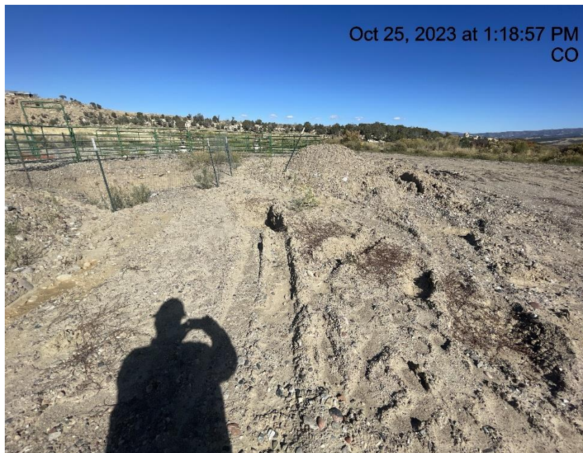
Photo # 4303 Lack of stabilization/compaction on location
