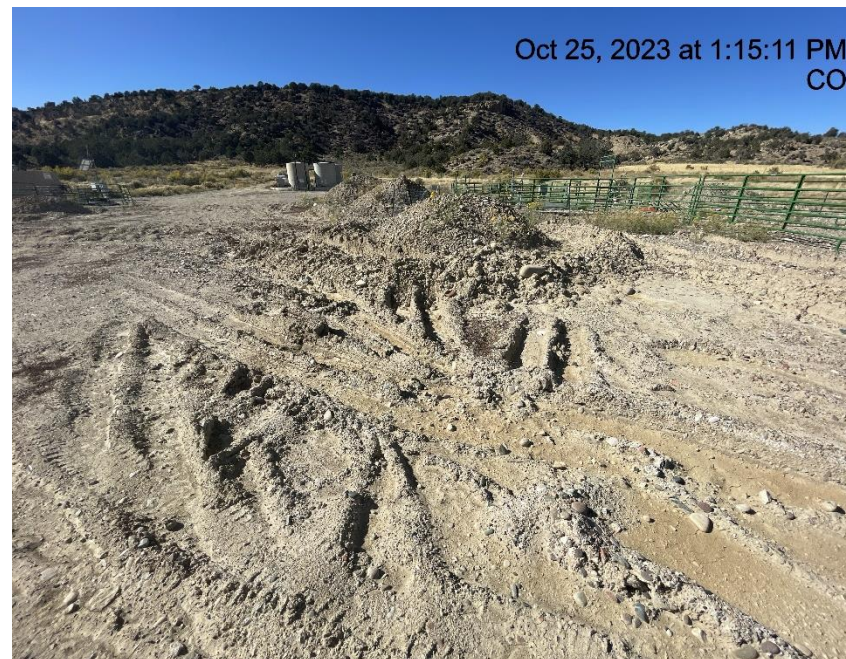
Photo # 4290 Lack of stabilization/compaction on location
