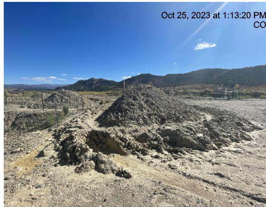
Photo # 4282 Vehicle tracks through berm around stockpiled soils/BMP needs maintenance
