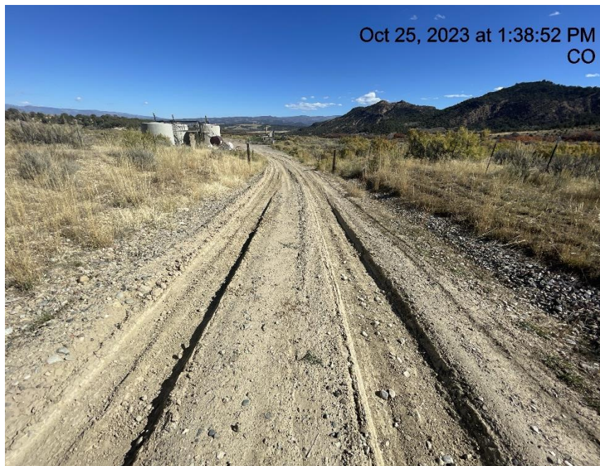
Photo # 4309 Lack of stabilization/compaction on lease road near entrance to location
