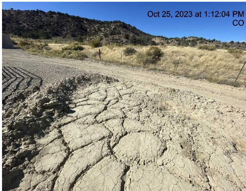
Photo # 4281 Berm around stockpiled soils has partially eroded/BMP needs maintenance
