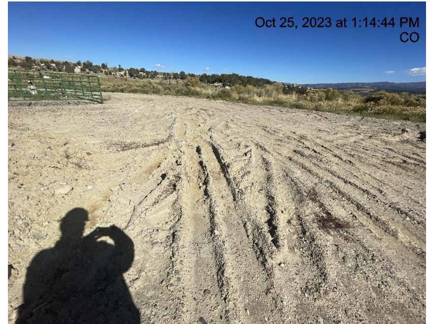
Photo # 4288 Lack of stabilization/compaction on location
