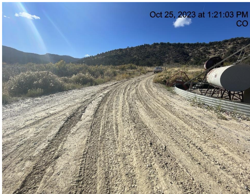
Photo # 4305 Lack of stabilization/compaction near entrance to location
