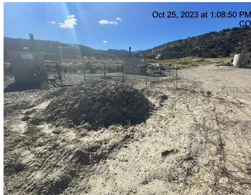
Photo # 4276 Berm around stockpiled soils has eroded/BMP needs maintenance
