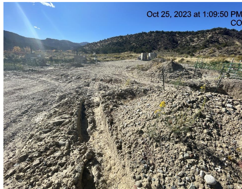
Photo # 4278 Vehicle tracks through berm around stockpiled soils/BMP needs maintenance
