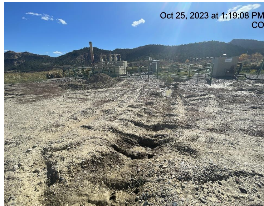
Photo # 4302 Lack of stabilization/compaction on location
