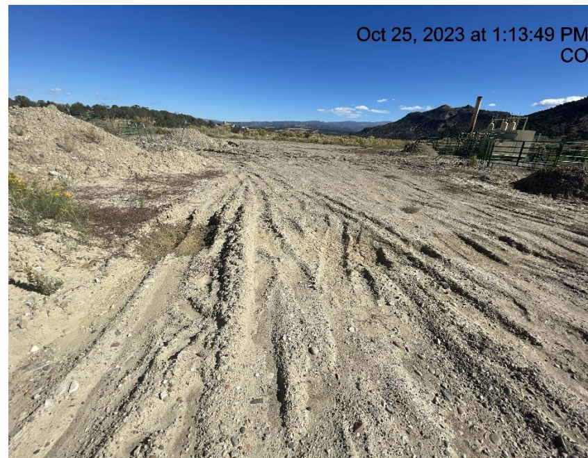
Photo # 4284 Lack of stabilization/compaction on location soils/BMP
