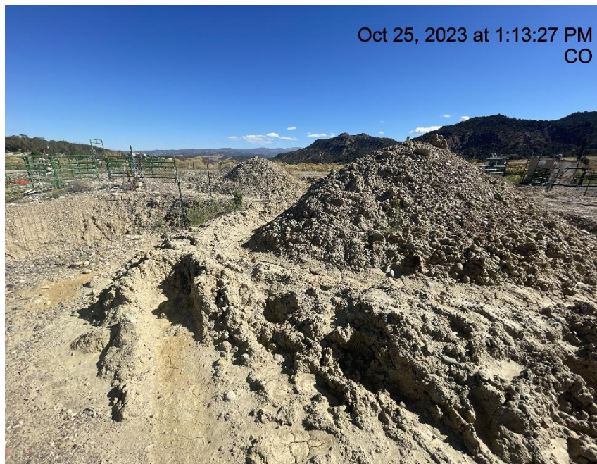
Photo # 4283 Vehicle tracks through berm around stockpiled soils/BMP needs maintenance
