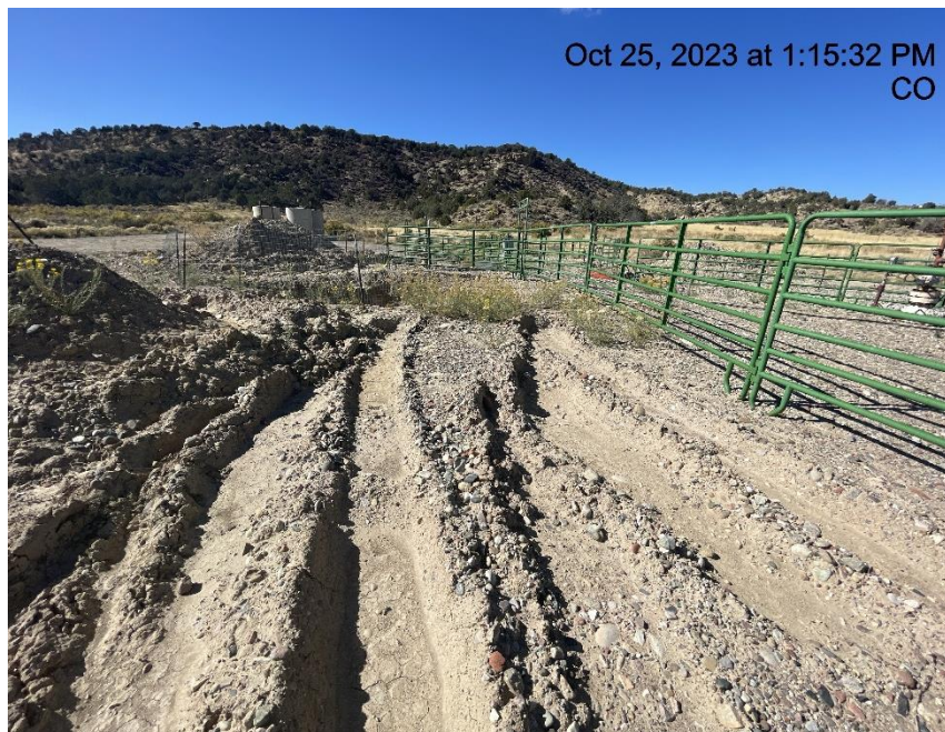
Photo # 4293 Lack of stabilization/compaction on location
