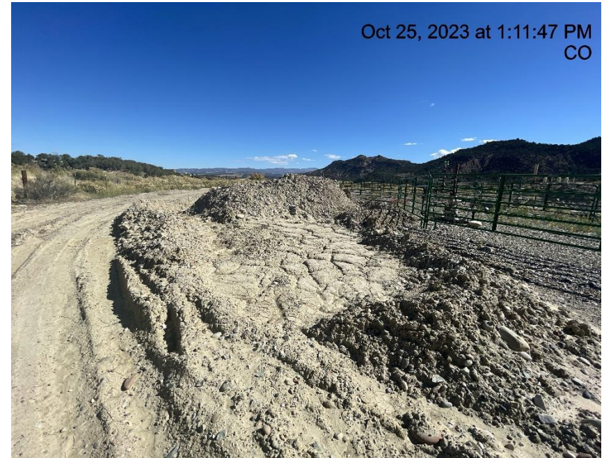
Photo # 4280 Berm around stockpiled soils has partially eroded/BMP needs maintenance
