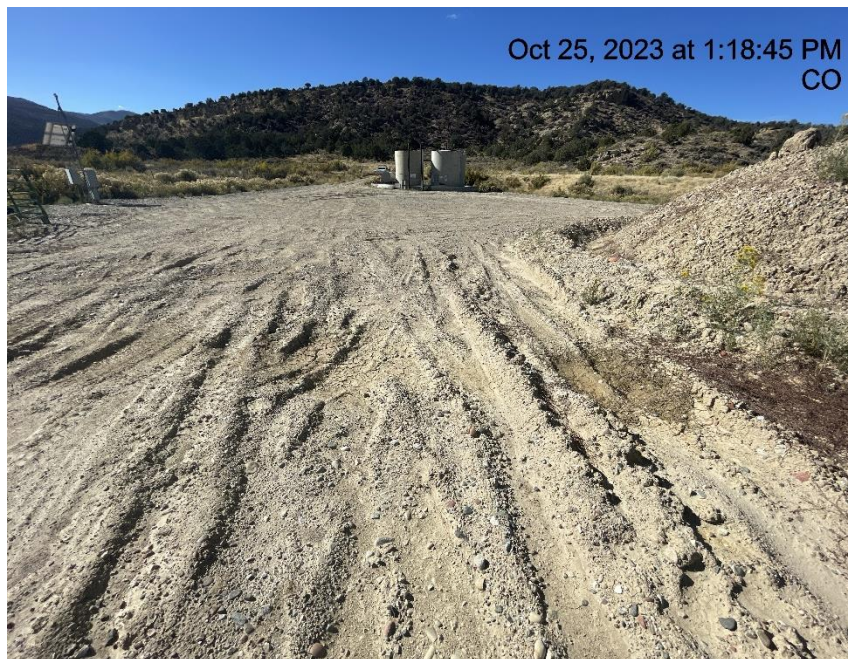
Photo # 4301 Lack of stabilization/compaction on location
