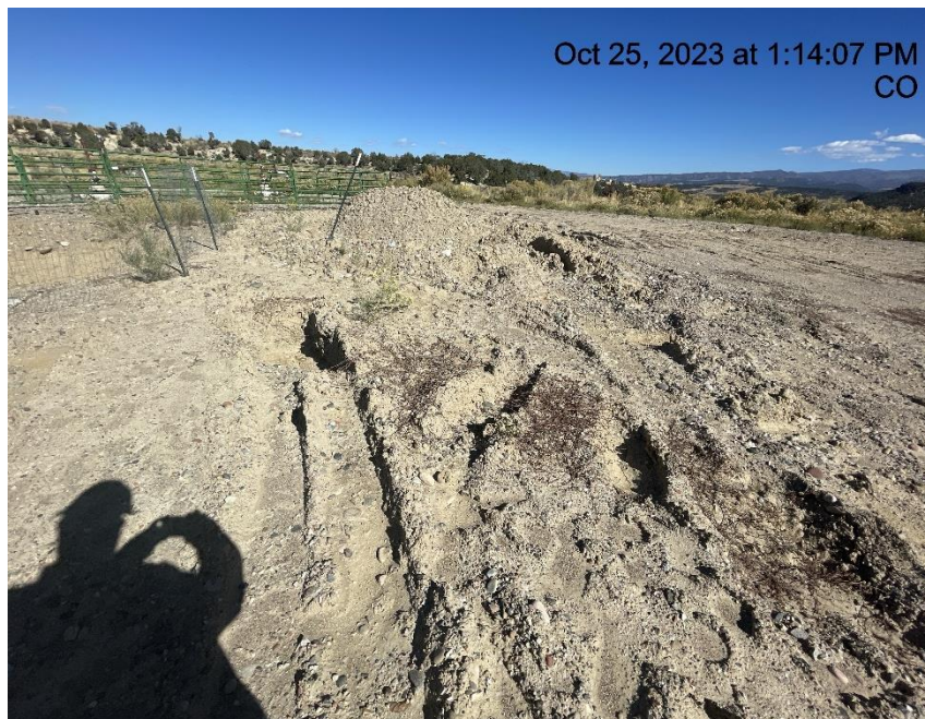
Photo # 4285 Lack of stabilization/compaction on location
