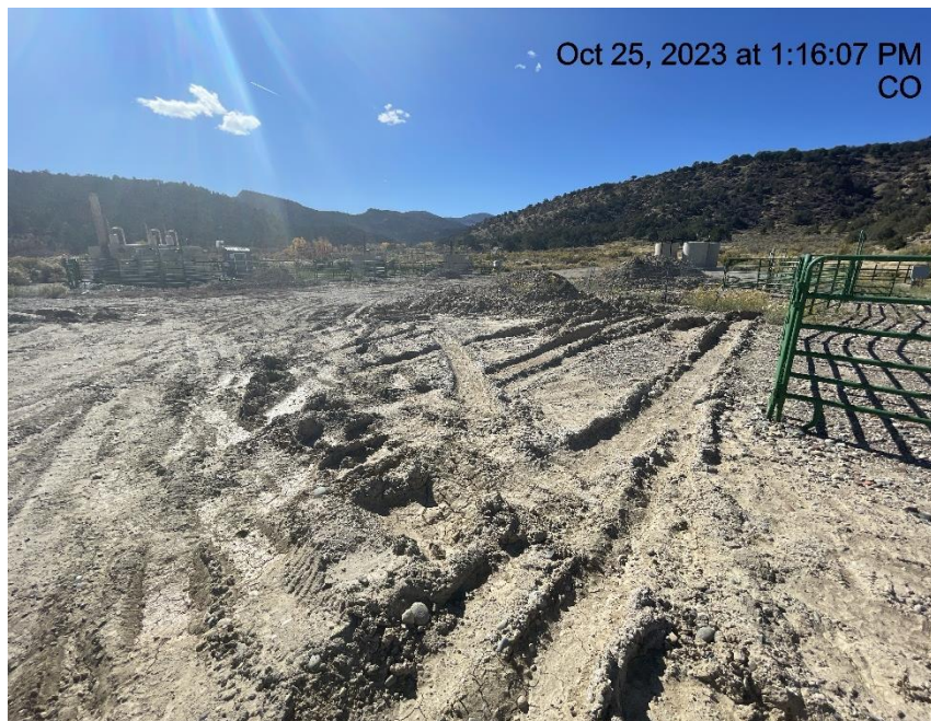
Photo # 4295 Lack of stabilization/compaction on location
