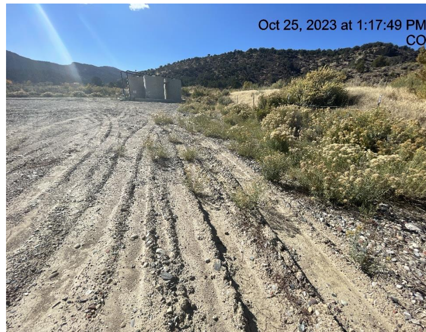
Photo # 4298 Lack of stabilization/compaction on location
