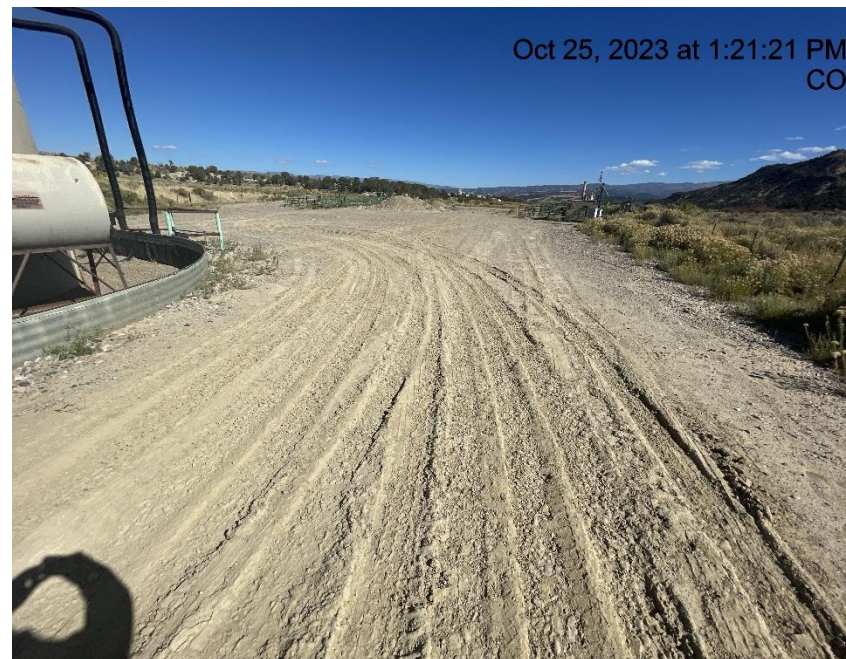
Photo # 4304 Lack of stabilization/compaction near entrance to location
