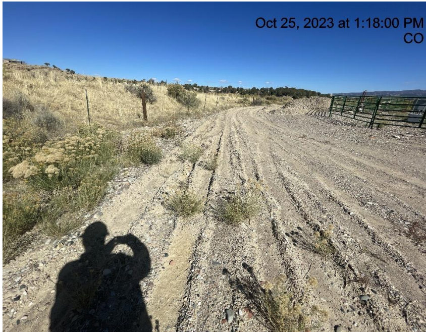
Photo # 4299 Lack of stabilization/compaction on location
