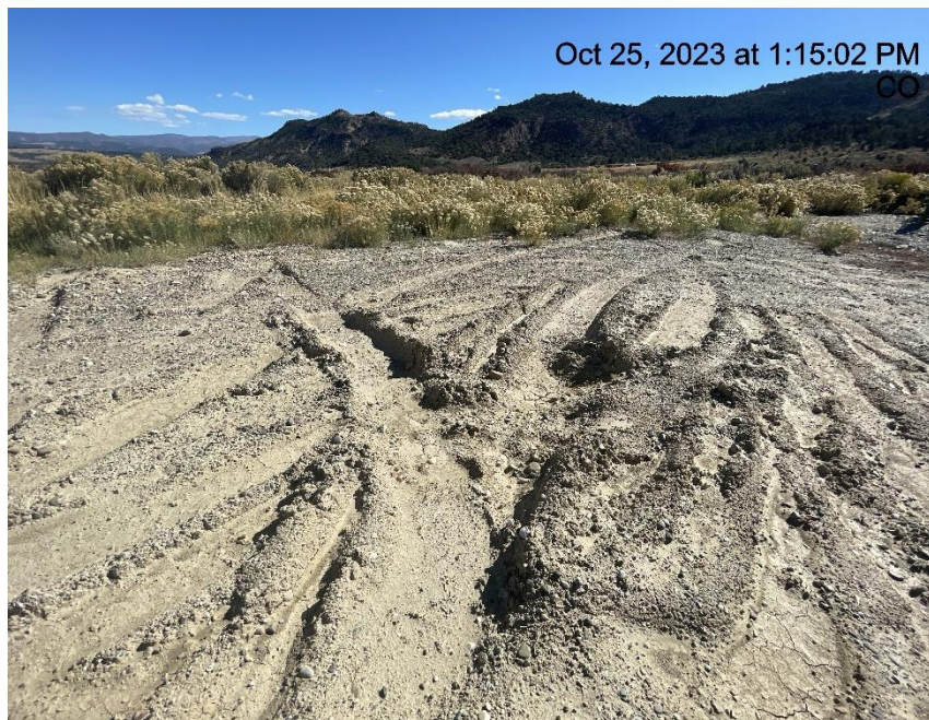
Photo # 4289 Lack of stabilization/compaction on location
