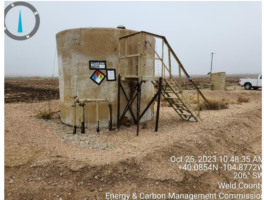
Photo 4 produced water tank and vacant 3" riser
