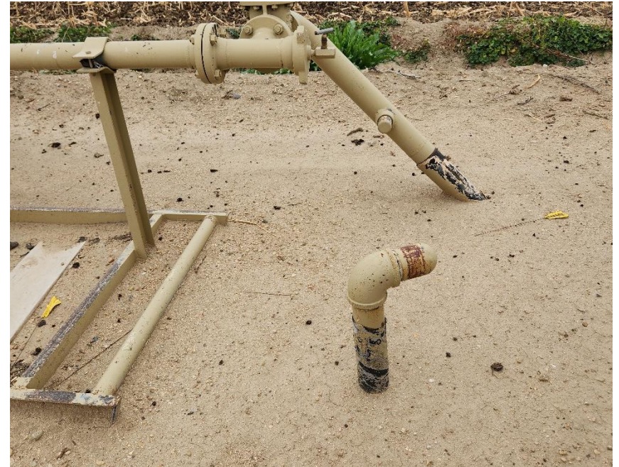
Photo 6 vacant 3" riser at meter run
