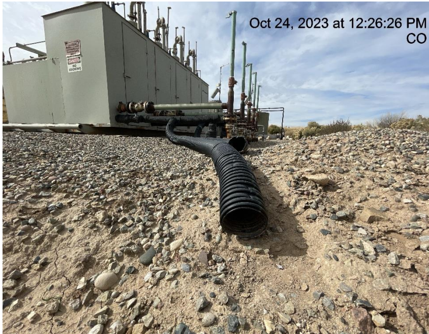
Photo # 4034 Flowline heating insulation open ended
