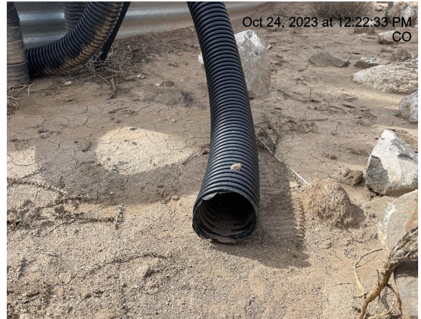
Photo # 4033 Flowline heating insulation open ended
