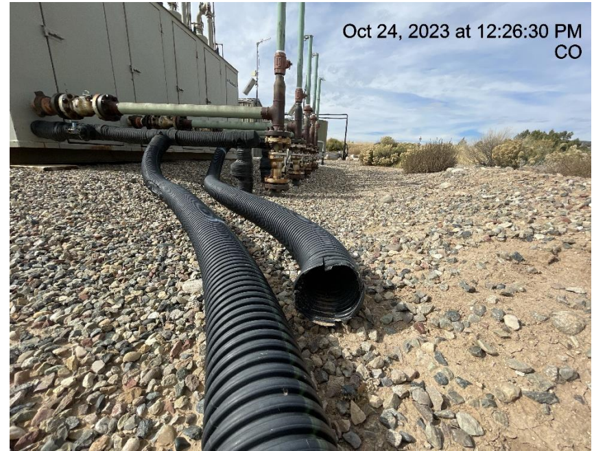
Photo # 4035 Flowline heating insulation open ended
