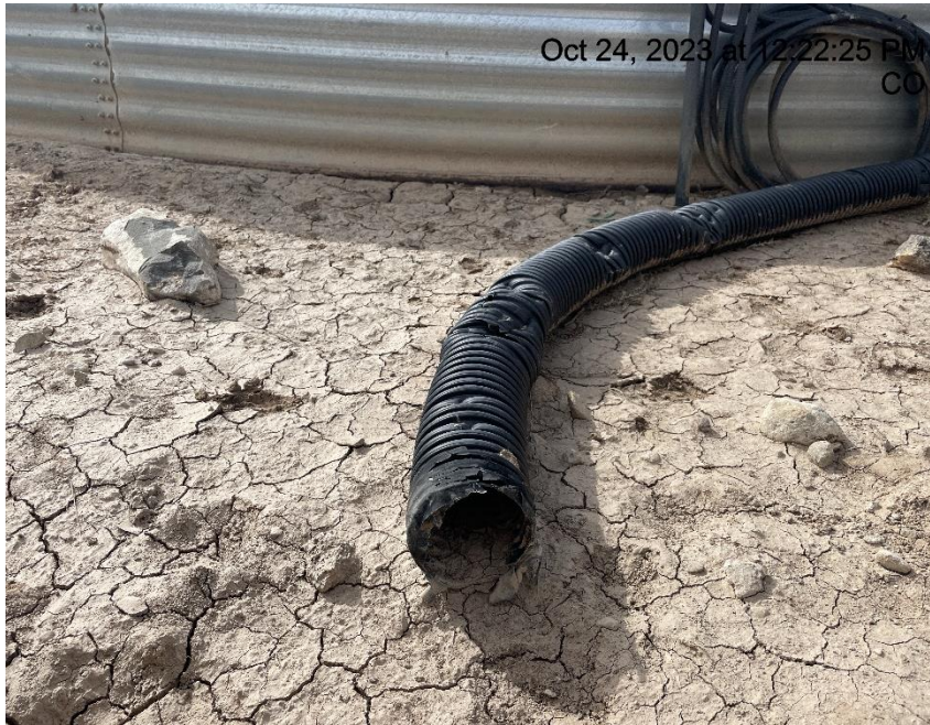
Photo # 4032 Flowline heating insulation open ended
