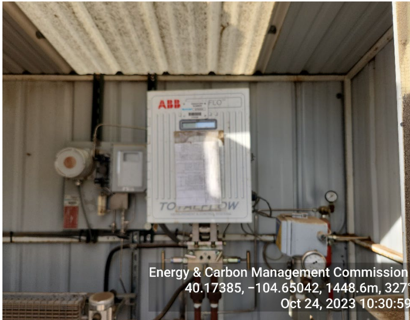
Photo 7: Disconnected gas meter
