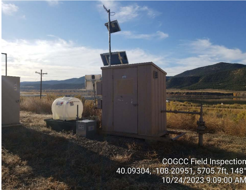
Photo #9 - Uncontrolled vegetation growth at gas meter shed
