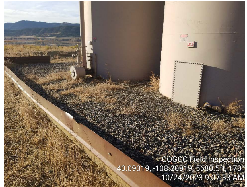
Photo #6 - Uncontrolled vegetation growth inside of tank battery secondary containment area (2).
