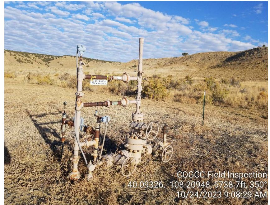
Photo #8 - Uncontrolled vegetation growth at wellhead.
