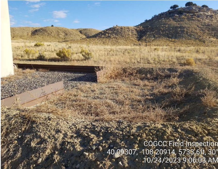
Photo #3 - Earthen berm on SE side of secondary containment area is eroded and overgrown.
