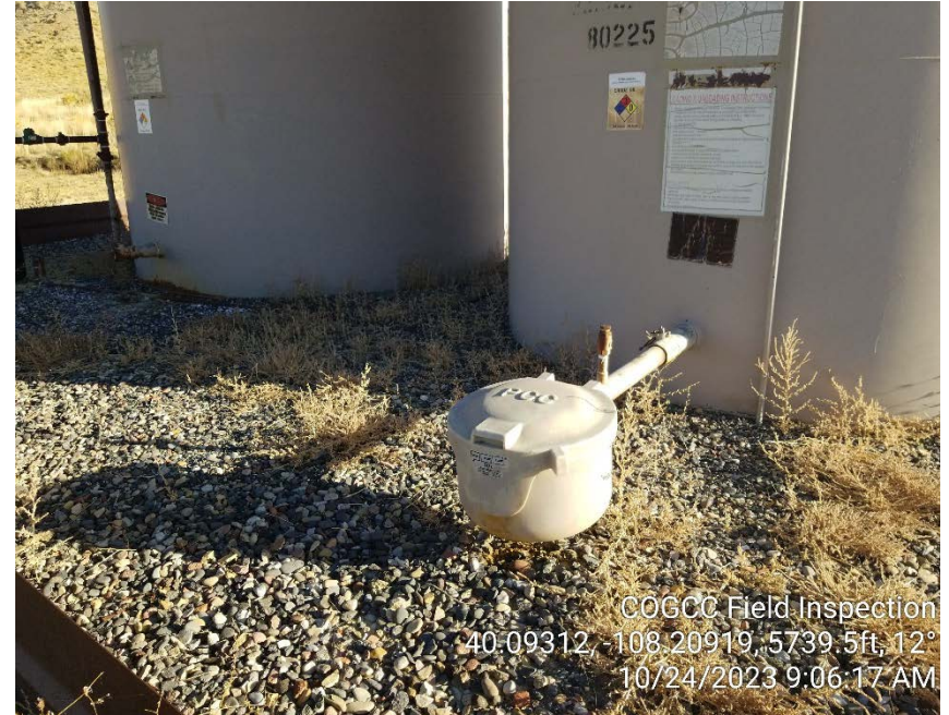
Photo #4 – Uncontrolled vegetation growth inside of tank battery secondary containment area (1).
