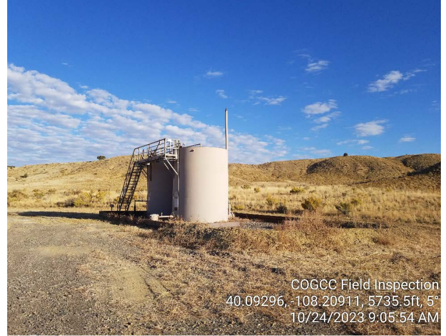
Photo #2 – View of tank battery from SE. Desktop calculation of secondary containment area volume is approximately 250-350 bbls assuming 1800 square feet area and a height of 1-1.5 feet. Vegetative growth along base and berms indicates that the berm is permeable. No liner was observed in secondary containment area during inspection.
