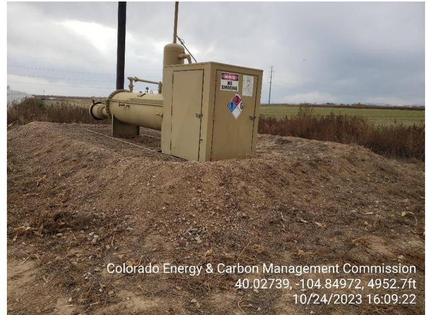
Photo 4 Horizontal Heated Separator.
