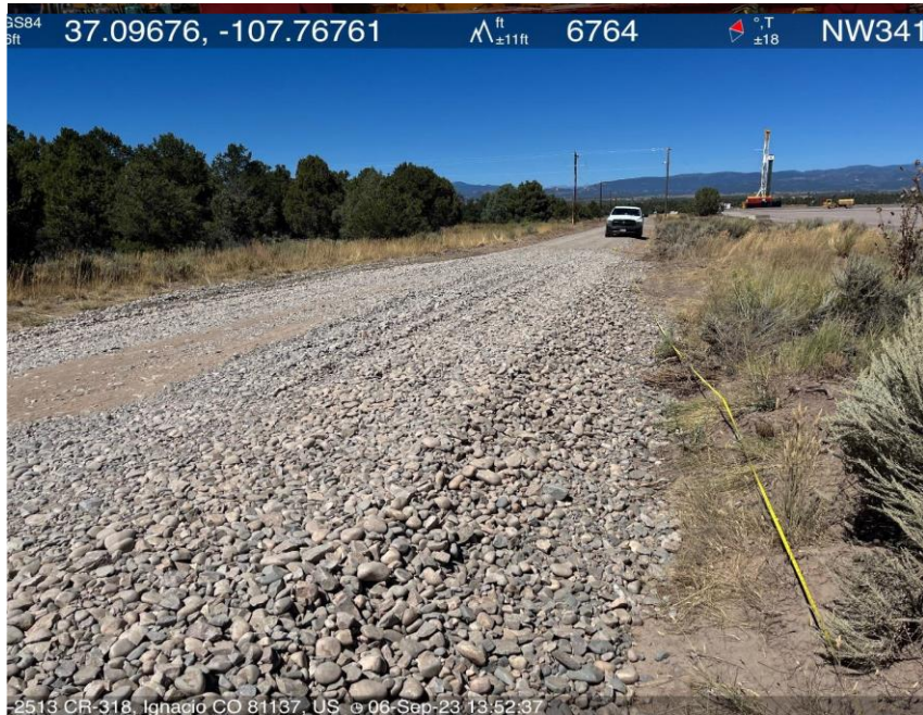
Photo #1 Tracking BMP installed during 9/8/2023 inspection.
