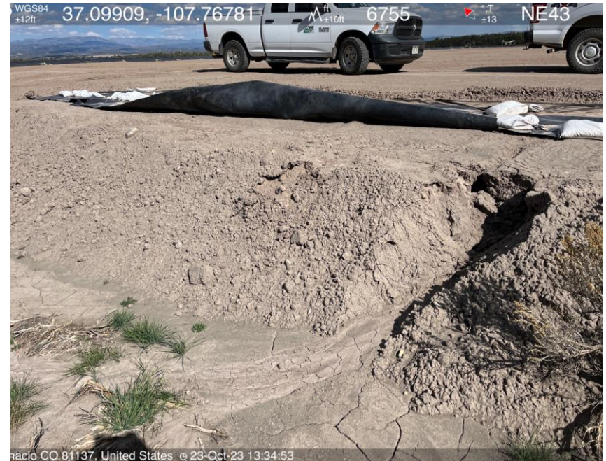
Photo #14 Gulley erosion at northwest entrance to tank pad.
