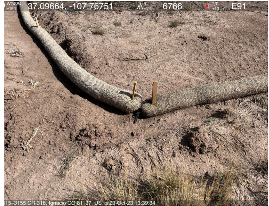
Photo #12 Wattle installation not to accepted specifications.
