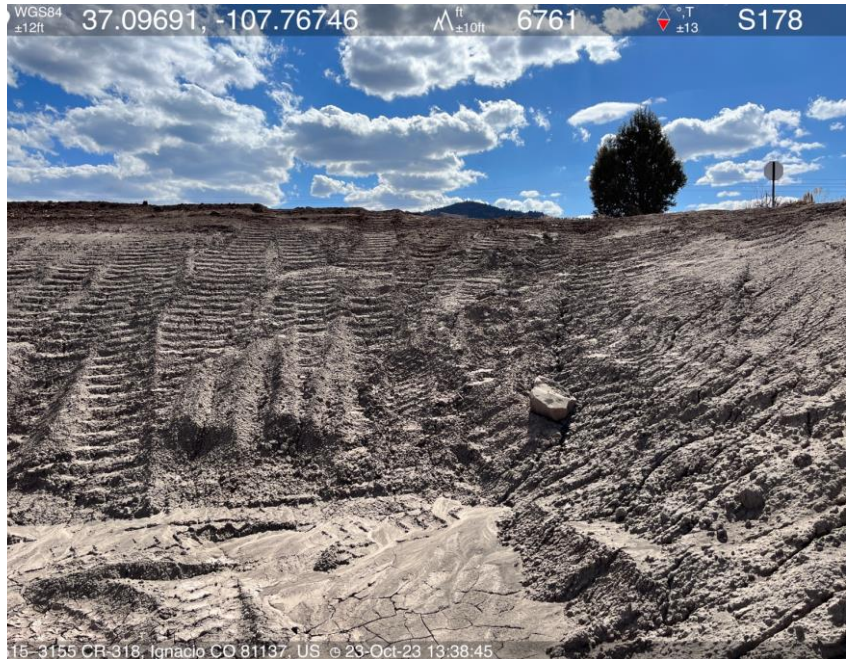
Photo #27 Vertical dozer tracking, however slopes not stabilized.
