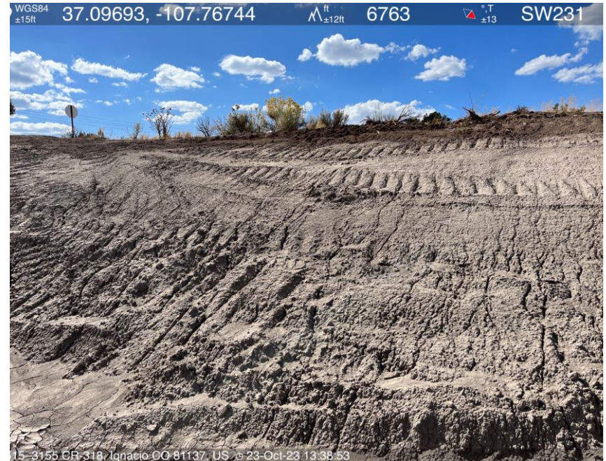
Photo #28 Horizontal dozer tracking, slopes not stabilized.
