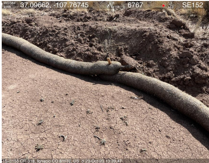
Photo #17 Wattle installation not to accepted specifications.
