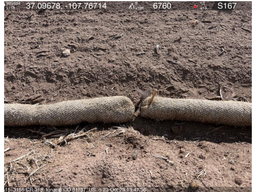
Photo #18 Wattle installation not to accepted specifications.
