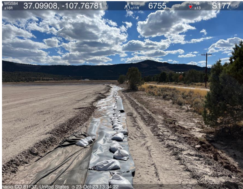
Photo #13 No perimeter wattles along west side of tank pad.
