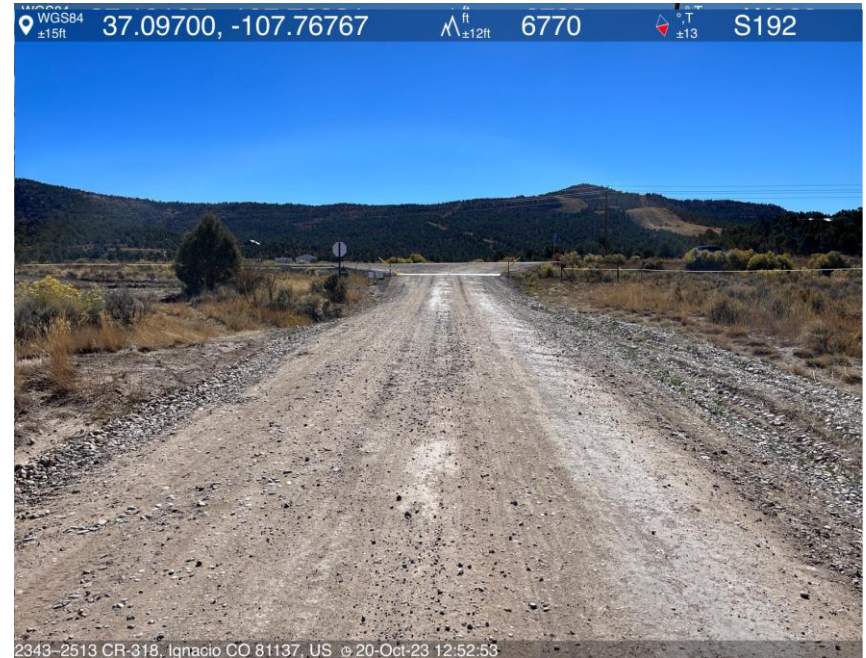
Photo #2 Tracking pad BMPs not maintained.
