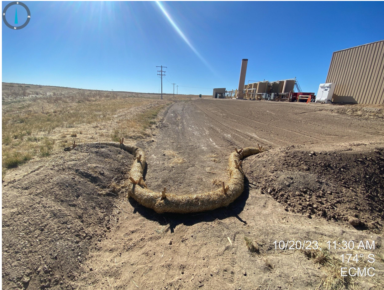
Photo 20. Taken from the southern portion of the sediment basin. Photo illustrates a temporary inlet control measure (e.g. straw wattle). More permanent control measures should be selected to provide long term stabilization.
