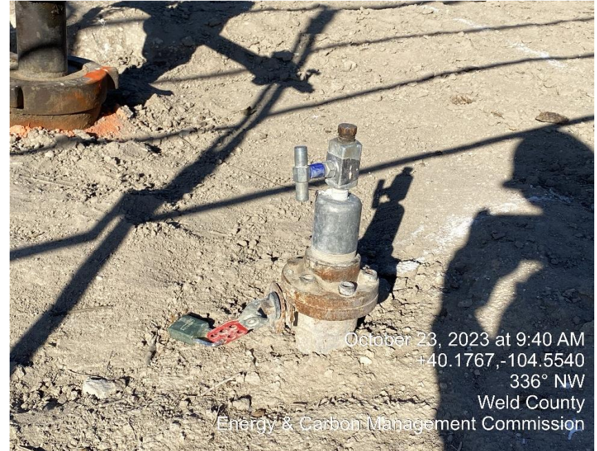
Riser needs tagged and identified
