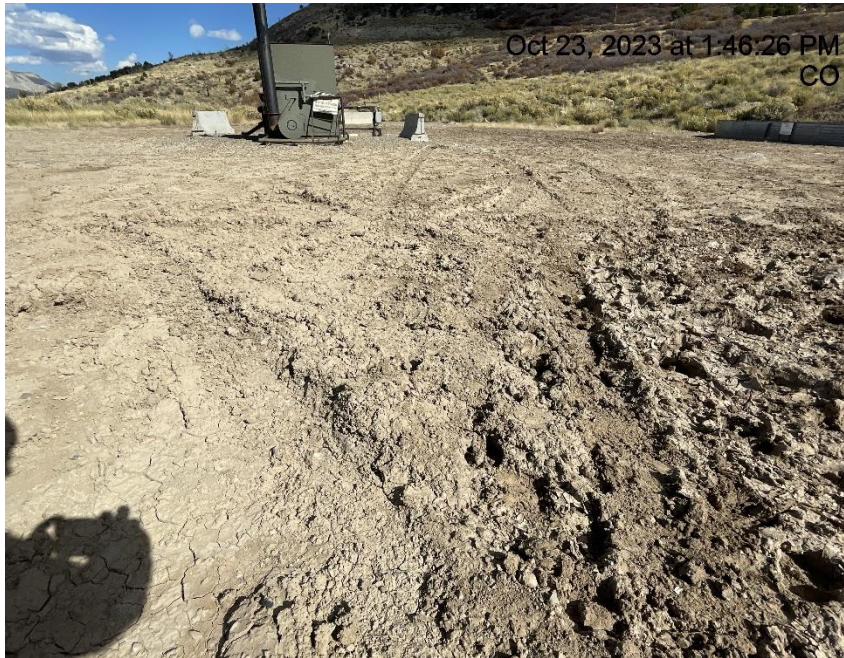
Photo # 3855 Lack of stabilization/compaction/insufficient tracking BMP's
