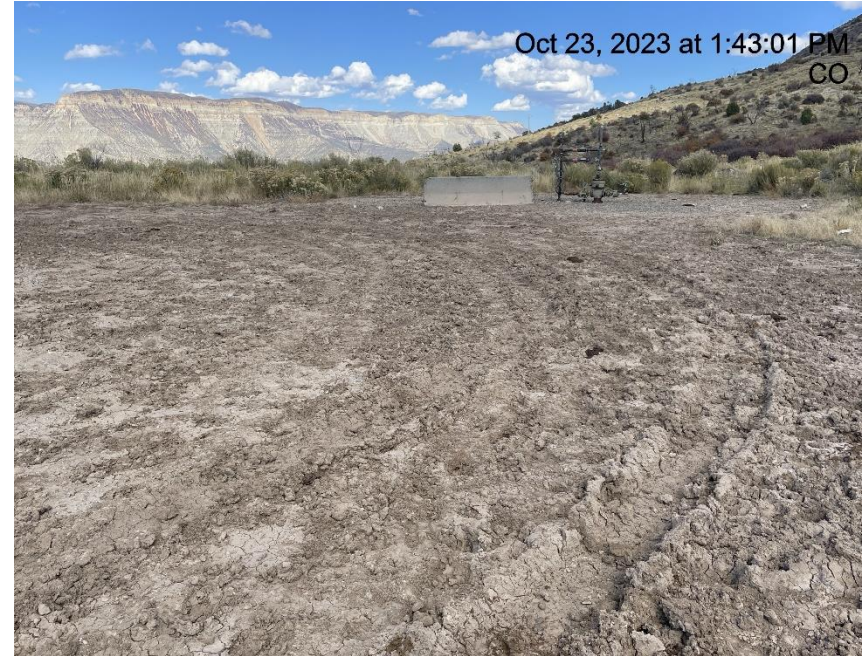
Photo # 3848 Lack of stabilization/compaction/insufficient tracking BMP's
