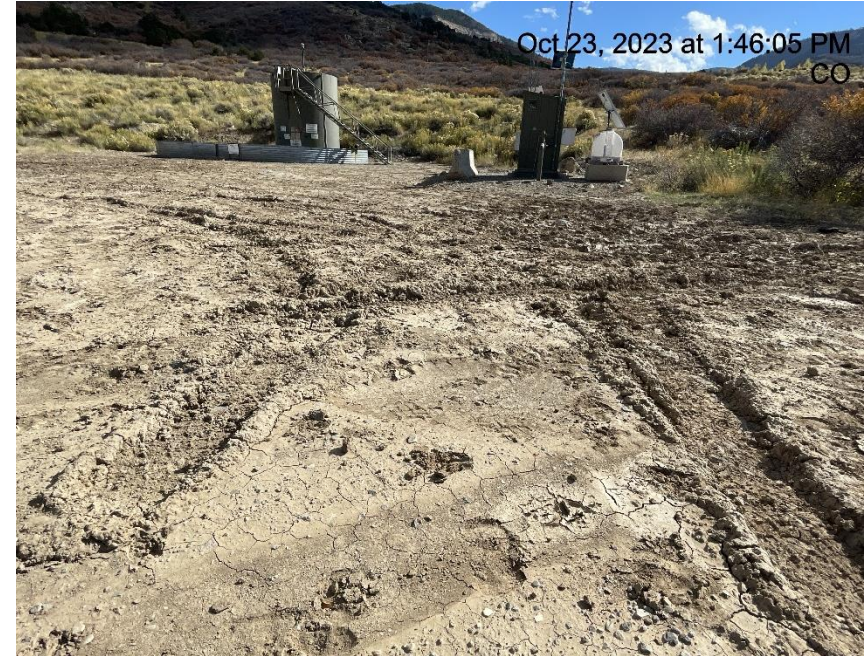
Photo # 3852 Lack of stabilization/compaction/insufficient tracking BMP's
