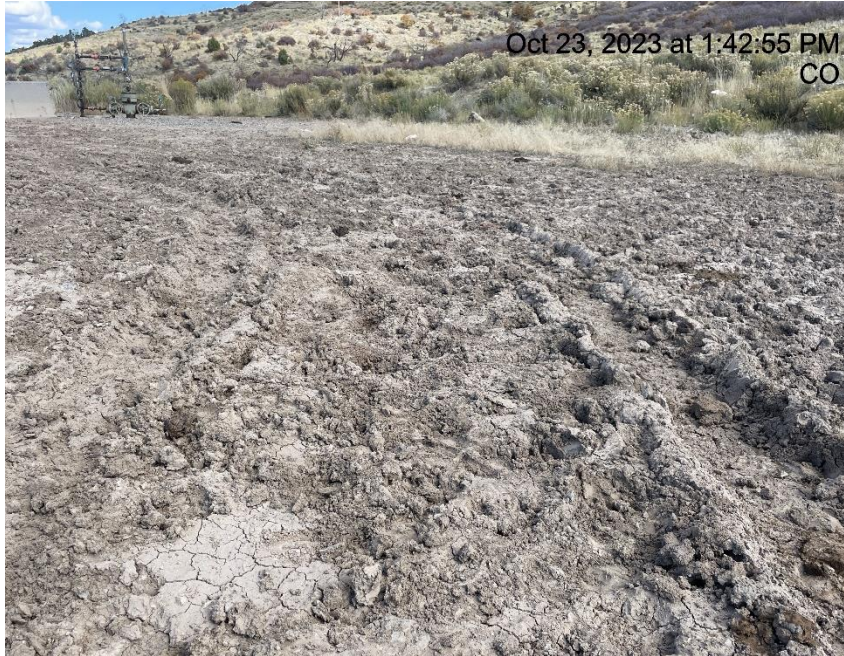
Photo # 3847 Lack of stabilization/compaction/insufficient tracking BMP's
