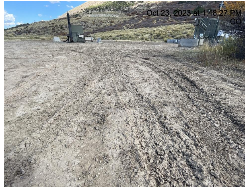
Photo # 3862 Lack of stabilization/compaction/insufficient tracking BMP's
