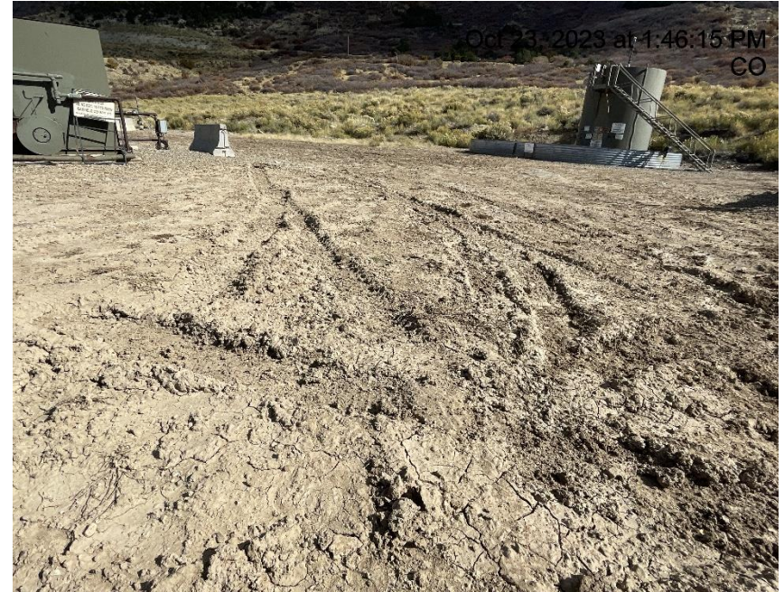
Photo # 3854 Lack of stabilization/compaction/insufficient tracking BMP's
