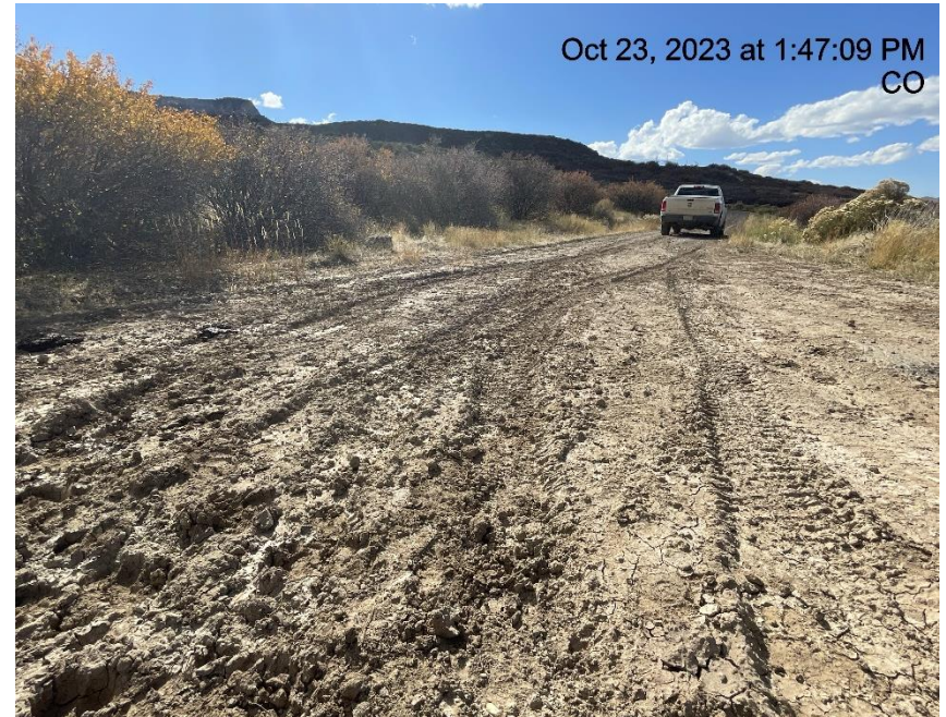
Photo # 3856 Lack of stabilization/compaction/insufficient tracking BMP's
