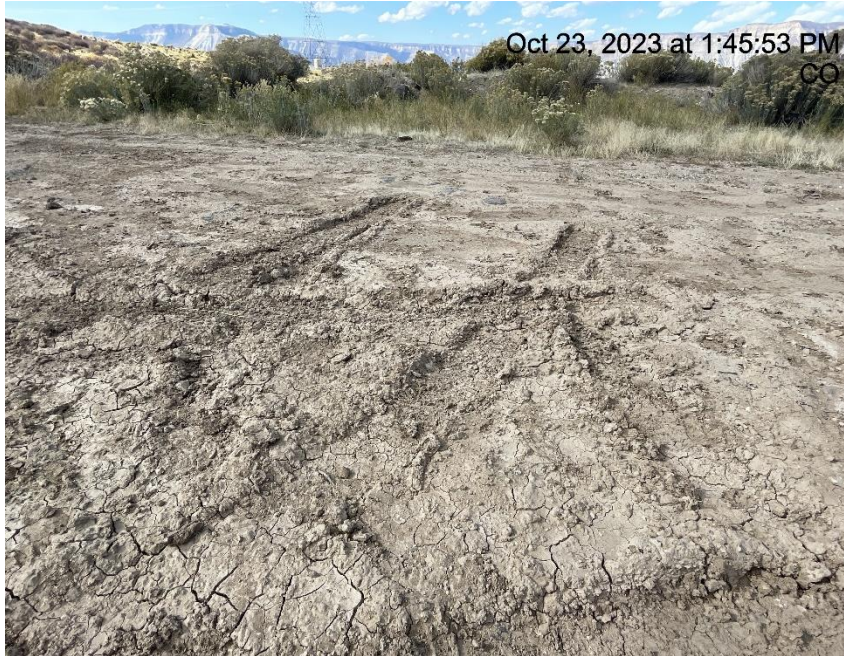
Photo # 3851 Lack of stabilization/compaction/insufficient tracking BMP's
