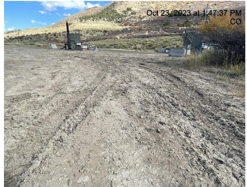
Photo # 3858 Lack of stabilization/compaction/insufficient tracking BMP's
