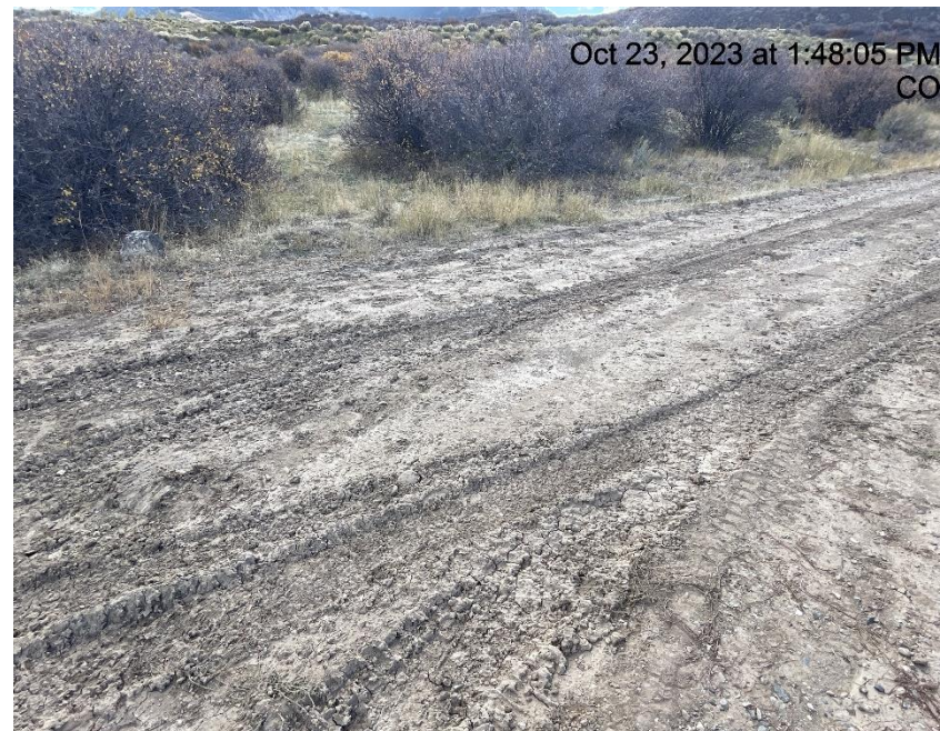
Photo # 3860 Lack of stabilization/compaction/insufficient tracking BMP's
