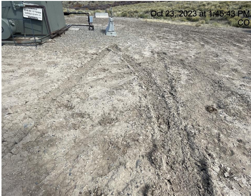
Photo # 3849 Lack of stabilization/compaction/insufficient tracking BMP's
