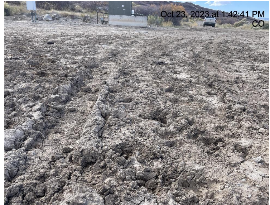
Photo # 3846 Lack of stabilization/compaction/insufficient tracking BMP's
