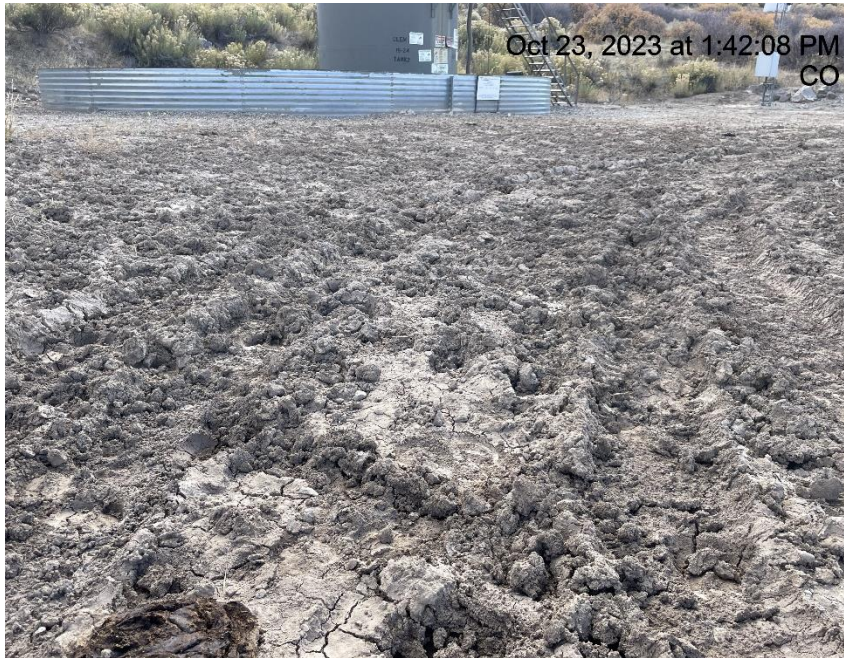
Photo # 3845 Lack of stabilization/compaction/insufficient tracking BMP's
