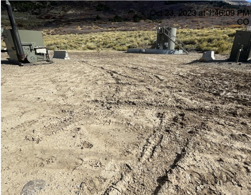
Photo # 3853 Lack of stabilization/compaction/insufficient tracking BMP's
