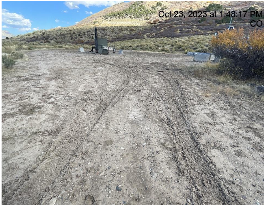
Photo # 3861 Lack of stabilization/compaction/insufficient tracking BMP's
