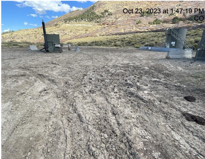
Photo # 3857 Lack of stabilization/compaction/insufficient tracking BMP's
