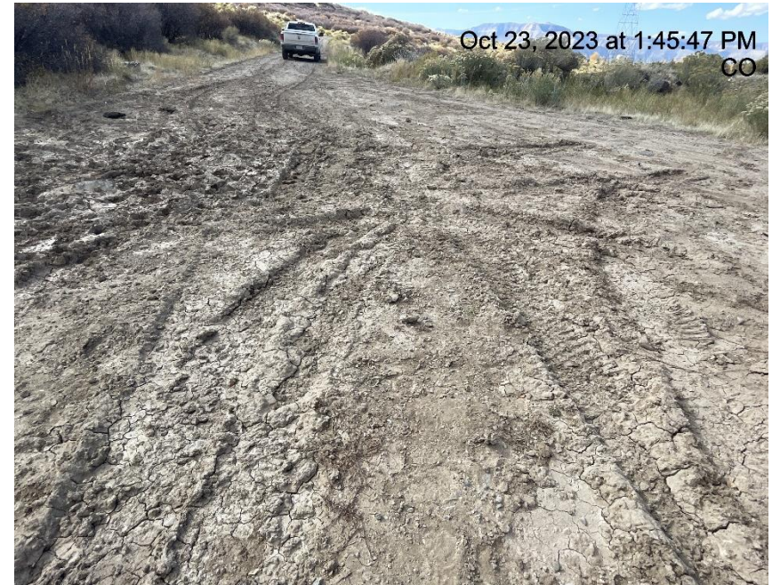
Photo # 3850 Lack of stabilization/compaction/insufficient tracking BMP's
