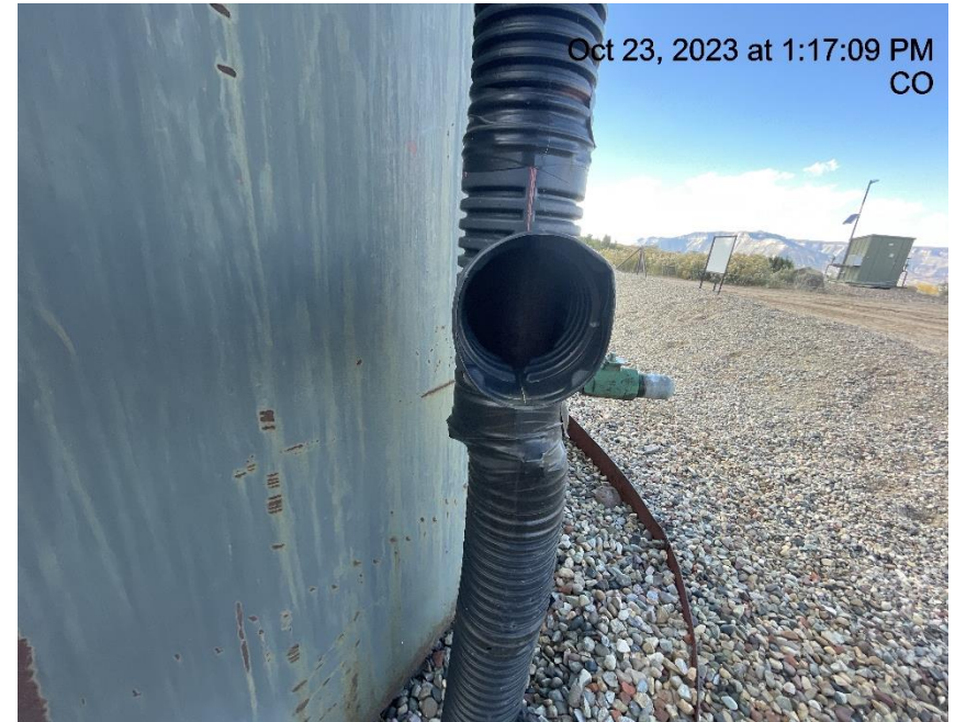
Photo # 3810 Flowline heating insulation open ended
