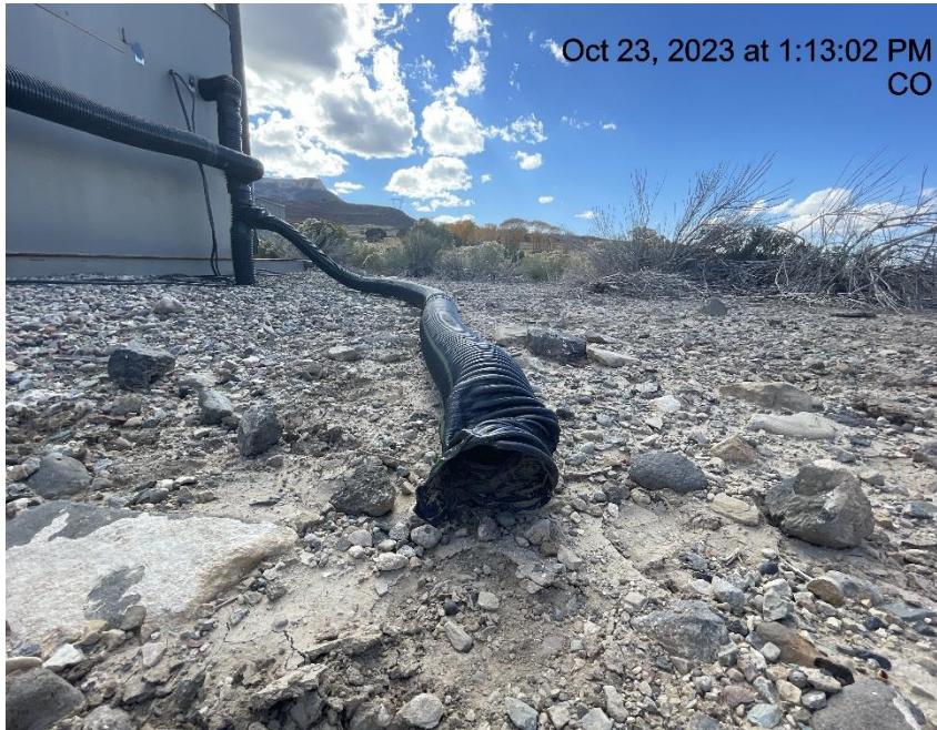
Photo # 3809 Flowline heating insulation open ended
