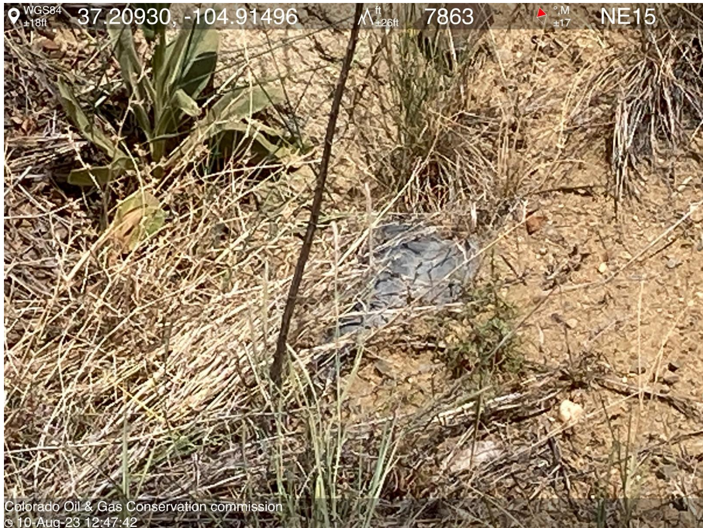
PHOTO 6: CULVERT APPROXIMATELY 200 YRD NORTH/ NORTHEAST OF LOCATION IS ALMOST COMPLETELY COVERED BY SEDIMENT. CLEAN AND MAINTAIN ALL CULVERTS ALONG ROW ACCORDING TO RULE 1002. CA DATE 9-10/2023.
