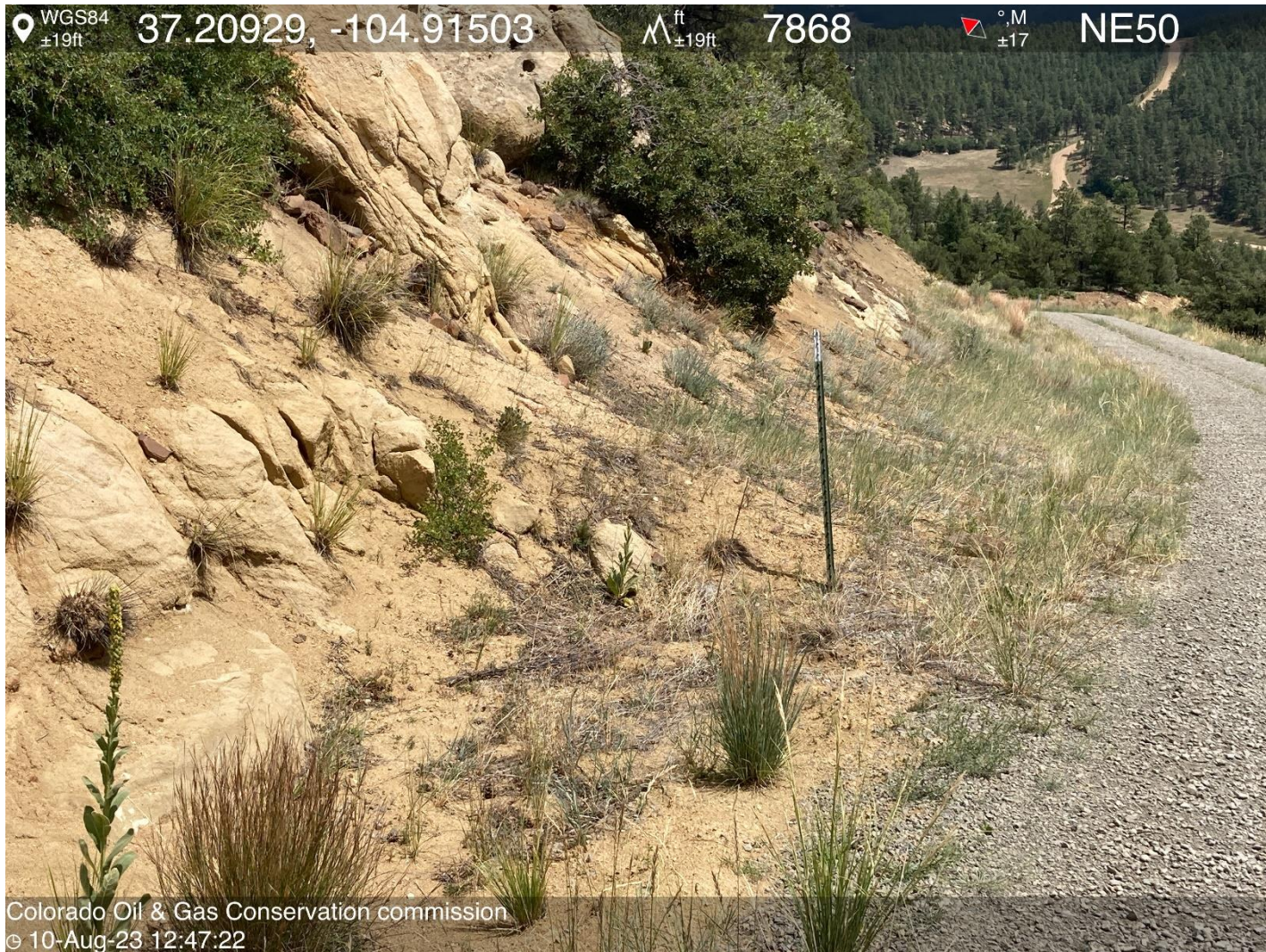
PHOTO 5: CULVERT JUST NORTH OF LOCATION IS ALMOST COMPLETELY COVERED BY SEDIMENT. CLEAN AND MAINTAIN ALL CULVERTS ALONG ROW ACCORDING TO RULE 1002. CA DATE 9-10/2023.
