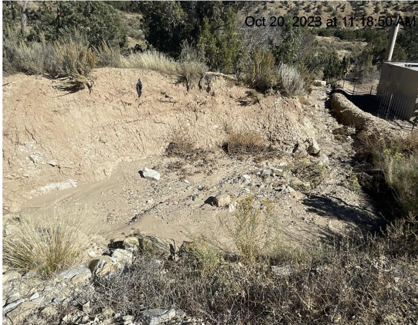
Photo # 3660 Sediment trap needs maintenance (W/NW area of location)
