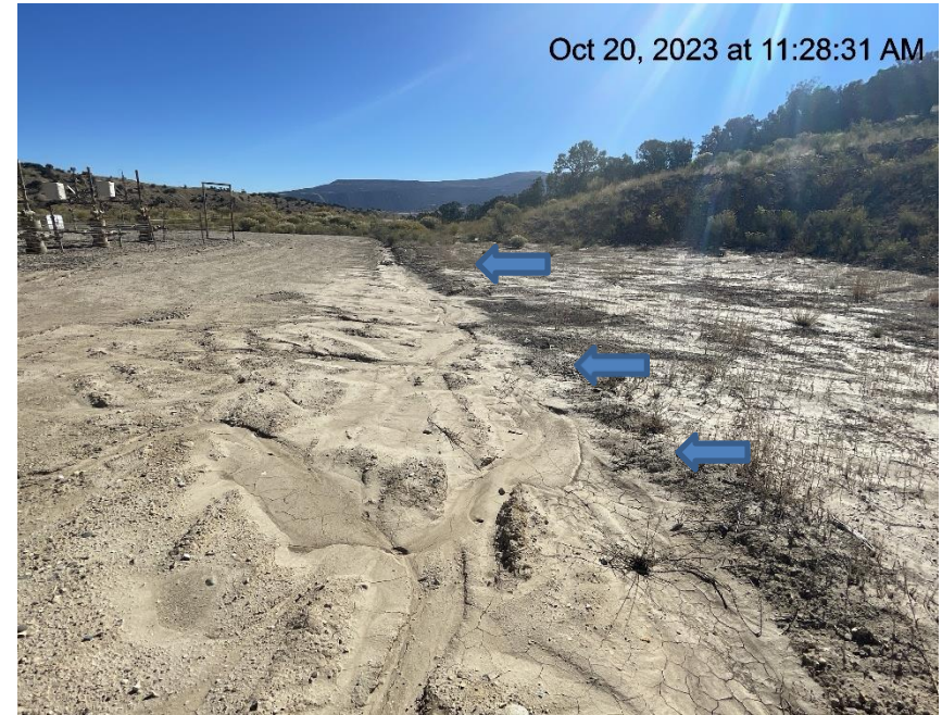
Photo # 3665 Ditch needs maintenance
