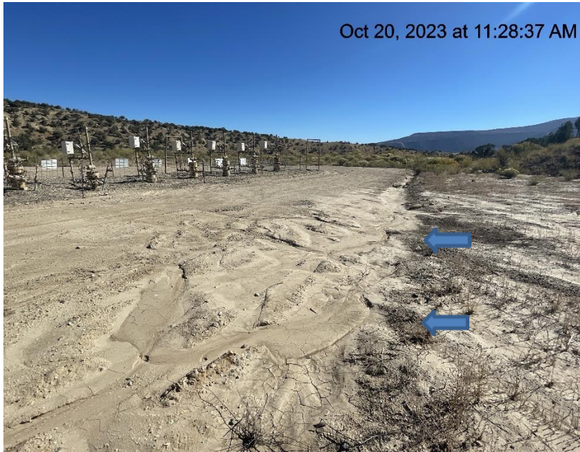
Photo # 3666 Ditch needs maintenance
