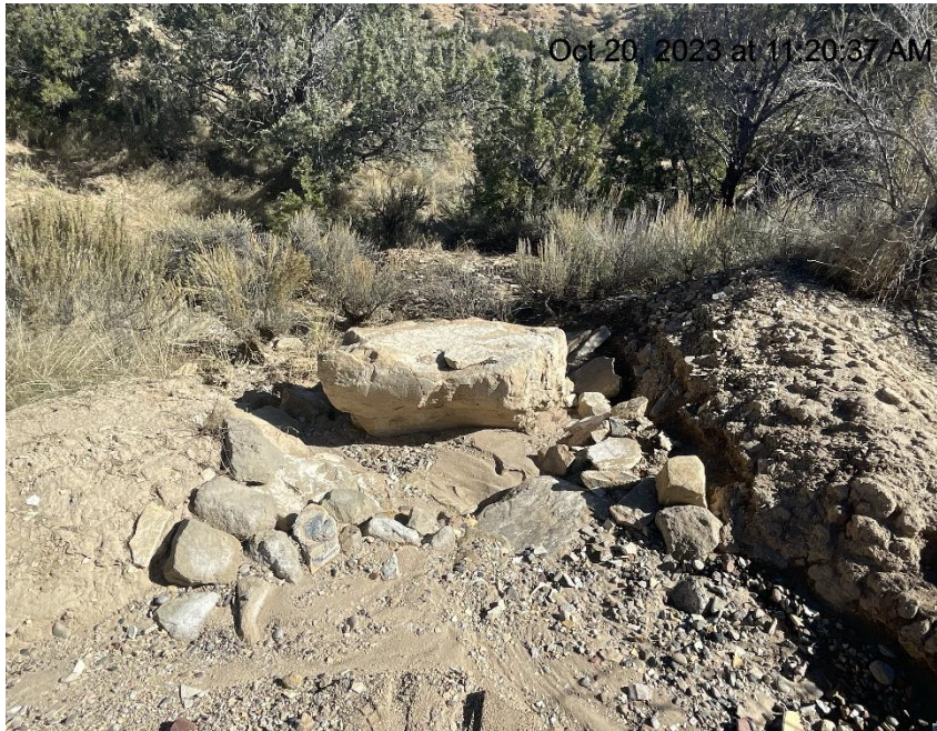
Photo # 3664 Sediment trap needs maintenance (NW corner of location)
