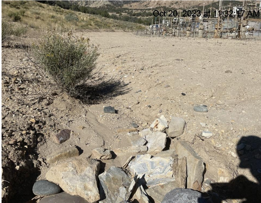
Photo # 3668 Check dam needs maintenance
