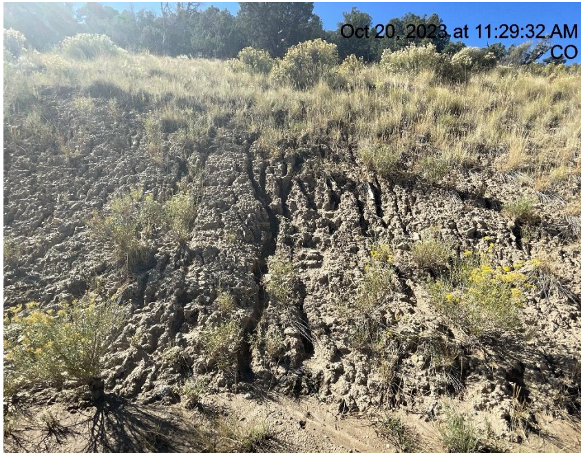
Photo # 3676 Erosion on slope & transport of sediment onto location (S/SE area of location)
