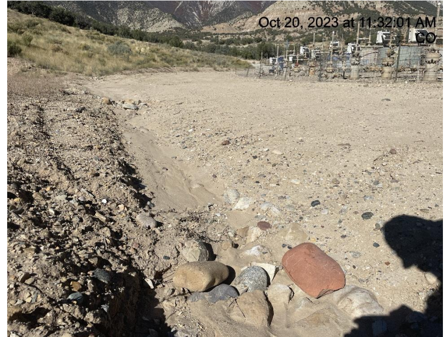
Photo # 3669 Check dam needs maintenance
