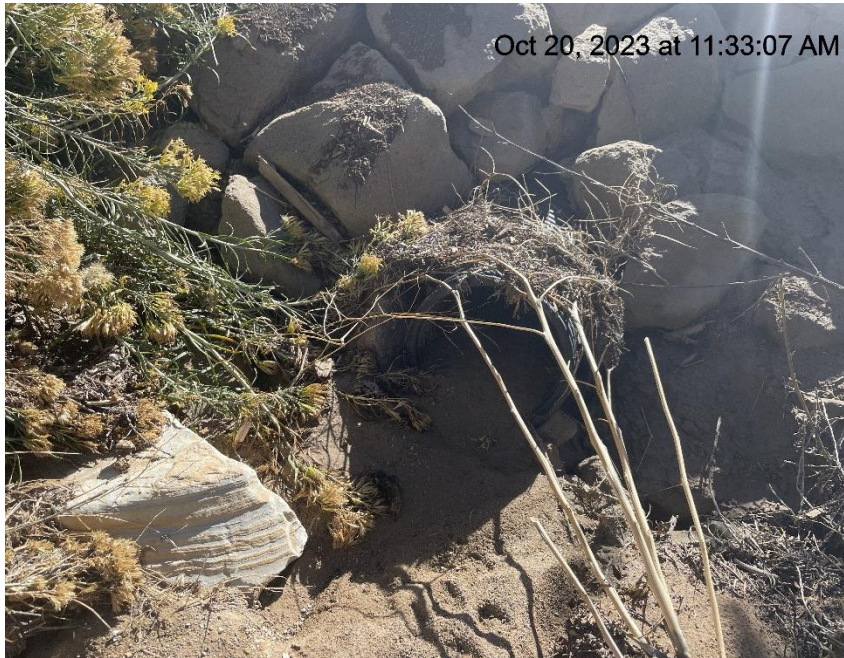
Photo # 3672 Sediment trap & drain need maintenance (SE corner of location)
