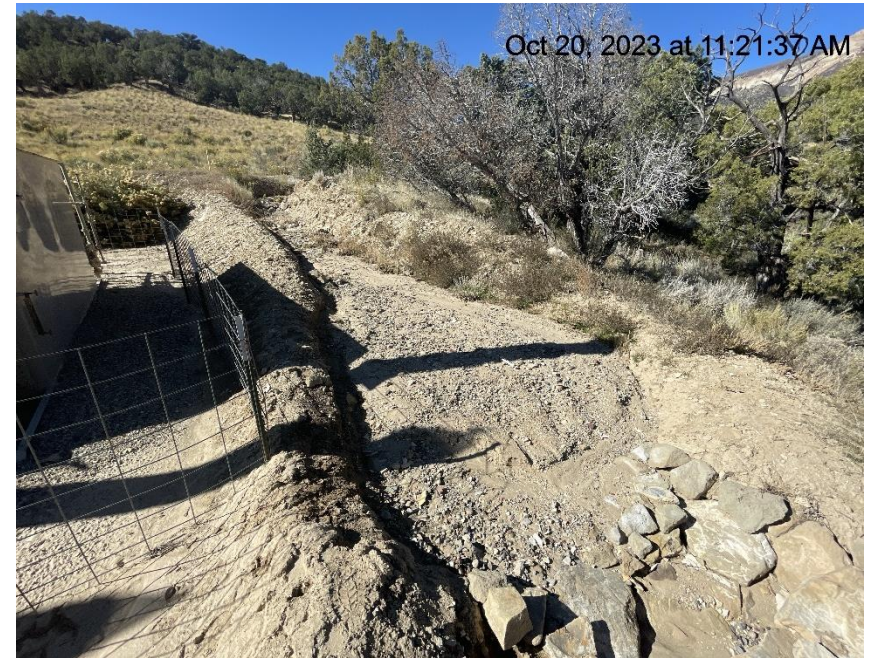
Photo # 3663 Sediment trap needs maintenance (NW corner of location)
