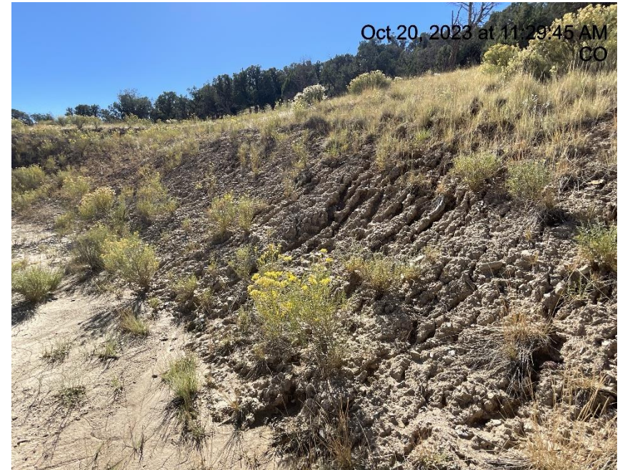
Photo # 3677 Erosion on slope & transport of sediment onto location (S/SE area of location)
