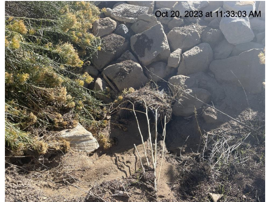
Photo # 3671 Sediment trap & drain need maintenance (SE corner of location)
