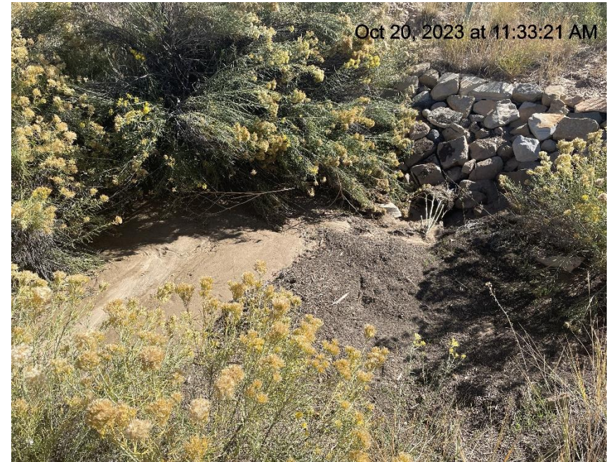
Photo # 3673 Sediment trap & drain need maintenance (SE corner of location)
