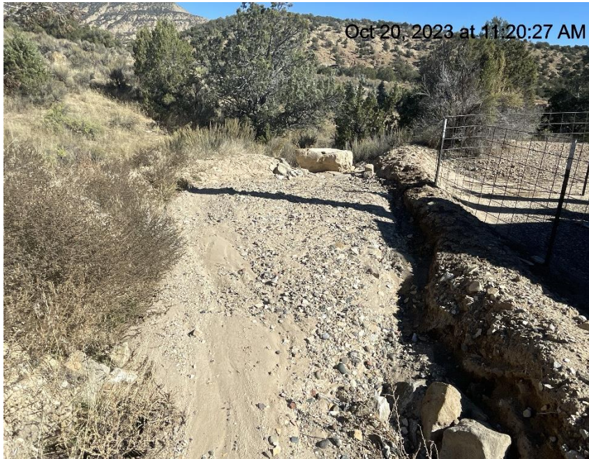
Photo # 3662 Sediment trap needs maintenance (NW corner of location)
