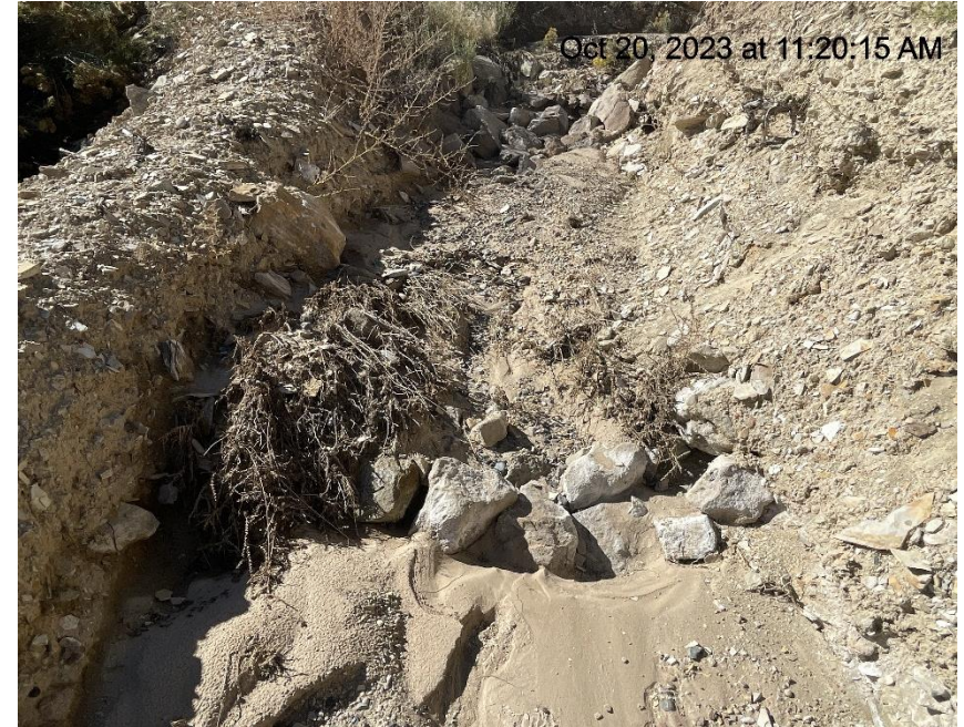
Photo # 3661 Check dam needs maintenance (W/NW area of location)
