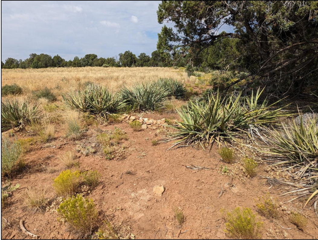
Photograph 7: View west of rock check dam in vegetated stormwater swale.
