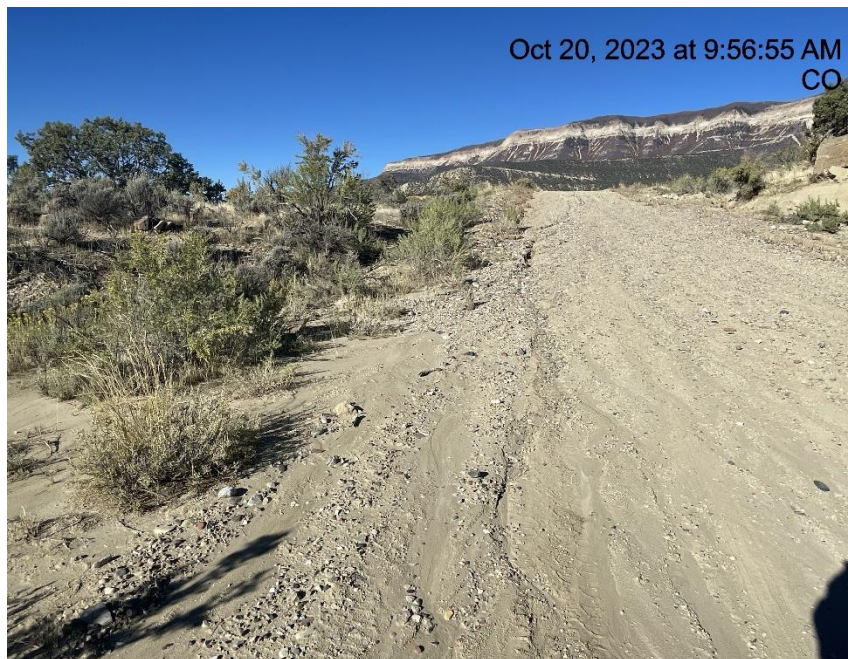
Photo # 3468 Erosion & transport of sediment off lease road into a vegetated area choking off vegetation/insufficient BMP's
