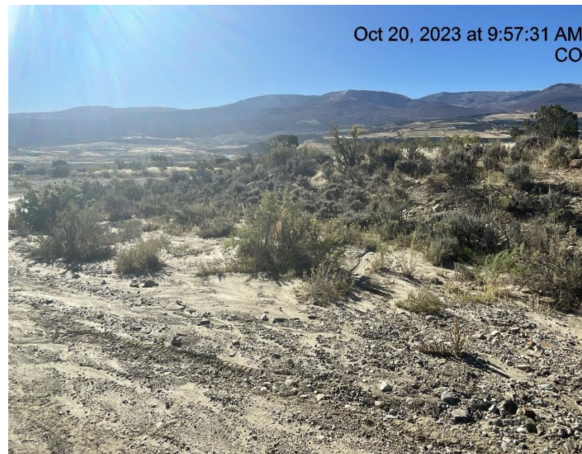
Photo # 3473 Erosion & transport of sediment off lease road into a vegetated area choking off vegetation/insufficient BMP's
