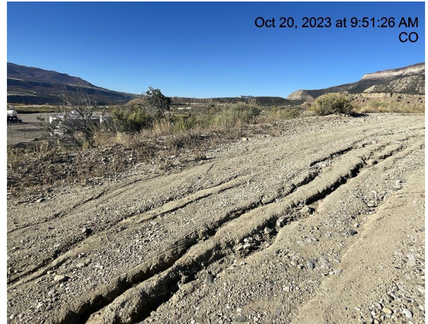
Photo # 3447 Erosion & transport of sediment on lease road /insufficient BMP's
