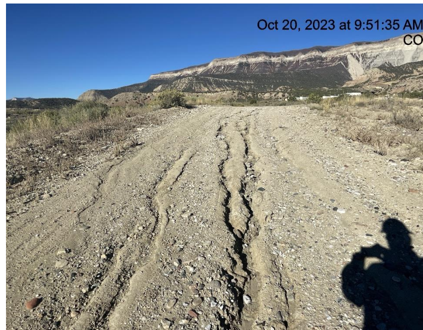
Photo # 3449 Erosion & transport of sediment on lease road /insufficient BMP's
