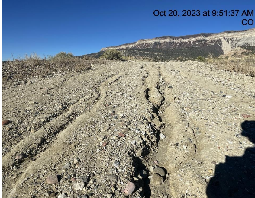
Photo # 3450 Erosion & transport of sediment on lease road /insufficient BMP's
