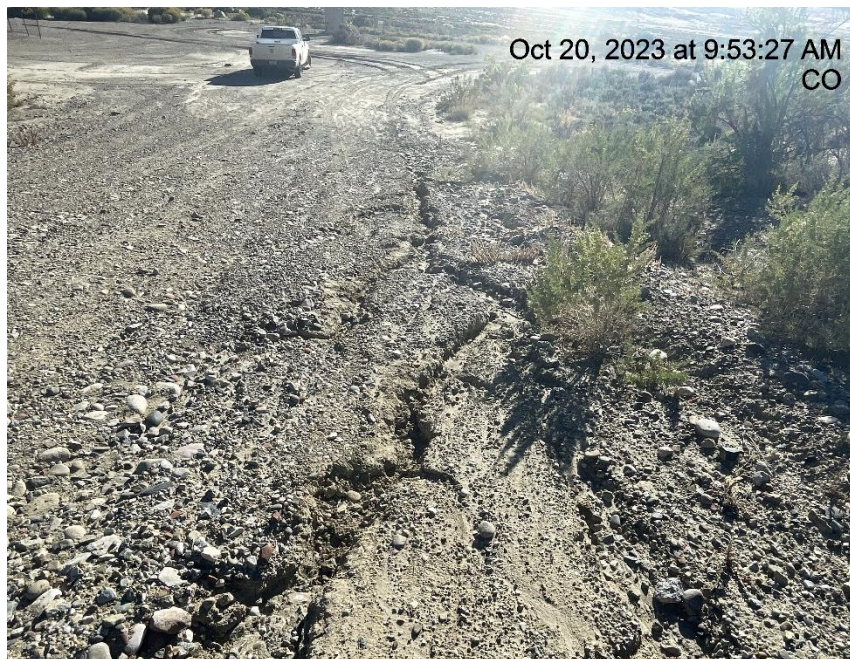
Photo # 3452 Erosion & transport of sediment off lease road into a vegetated area choking off vegetation/insufficient BMP's
