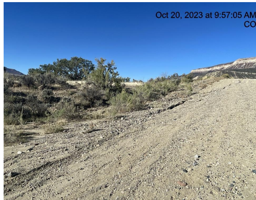
Photo # 3469 Erosion & transport of sediment off lease road into a vegetated area choking off vegetation/insufficient BMP's
