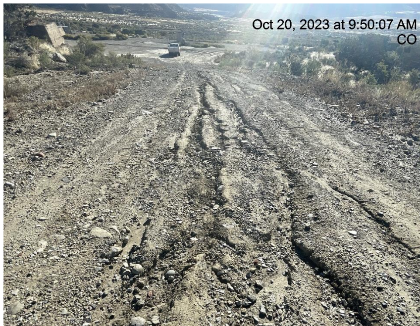
Photo # 3442 Erosion & transport of sediment off lease road into a vegetated area choking off vegetation/insufficient BMP's
