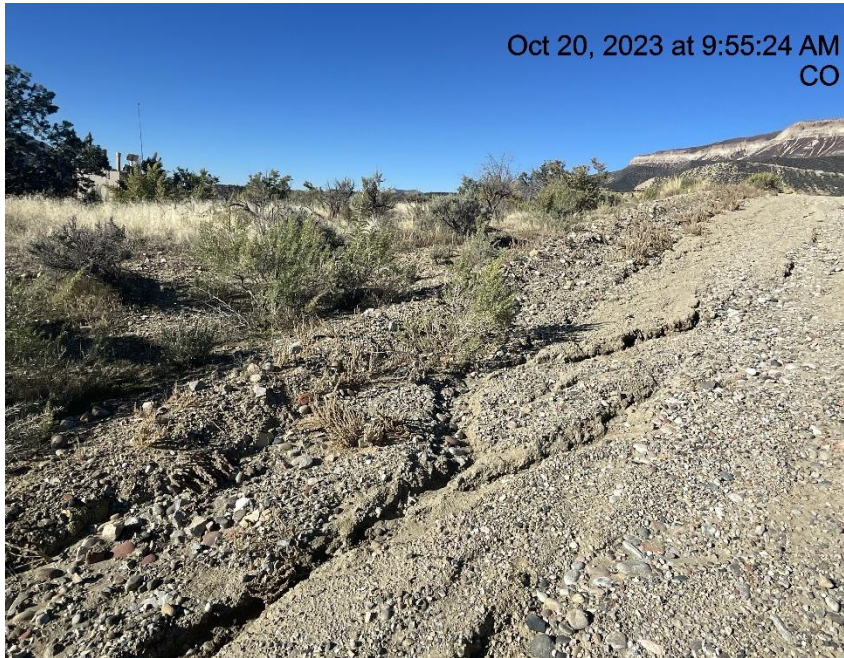
Photo # 3460 Erosion & transport of sediment off lease road into a vegetated area choking off vegetation/insufficient BMP's
