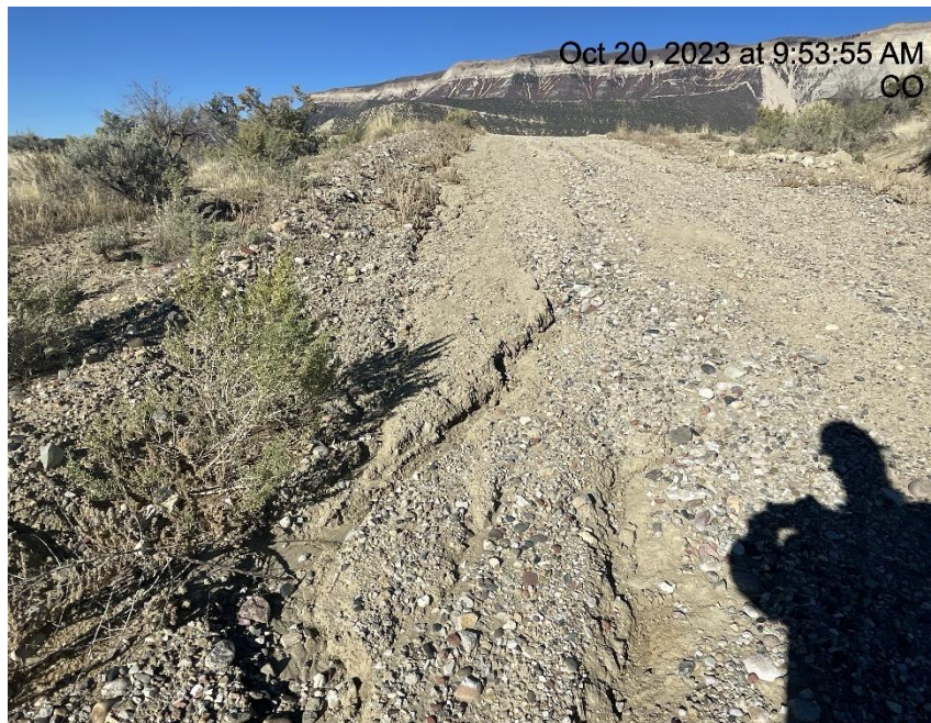
Photo # 3454 Erosion & transport of sediment off lease road into a vegetated area choking off vegetation/insufficient BMP's
