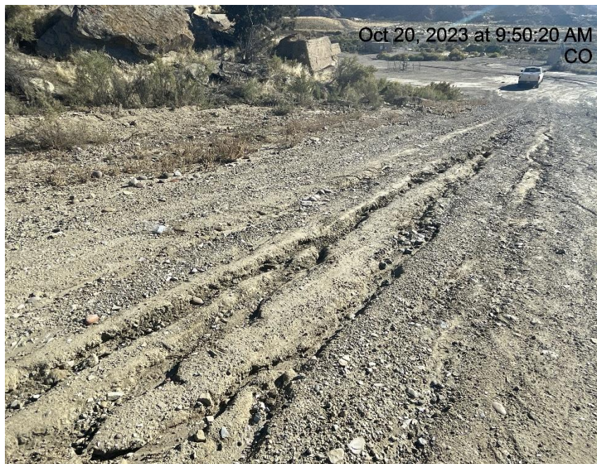
Photo # 3444 Erosion & transport of sediment on lease road /insufficient BMP's
