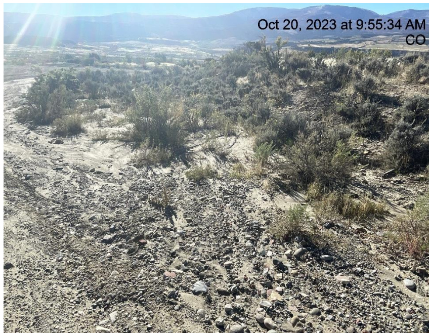
Photo # 3462 Erosion & transport of sediment off lease road into a vegetated area choking off vegetation/insufficient BMP's
