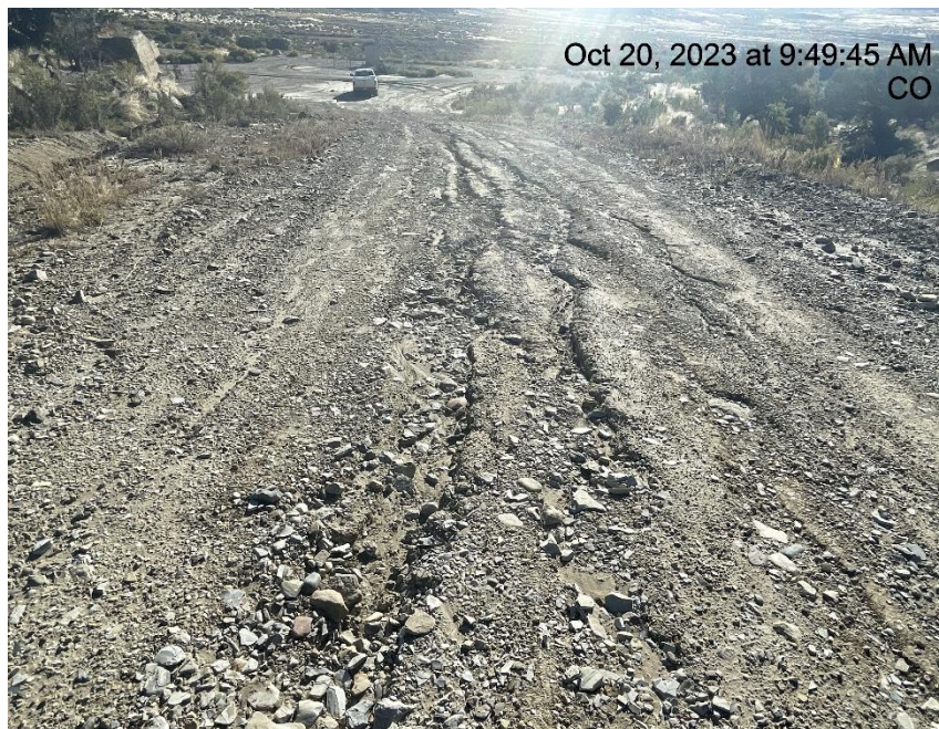
Photo # 3440 Erosion & transport of sediment on lease road /insufficient BMP's
