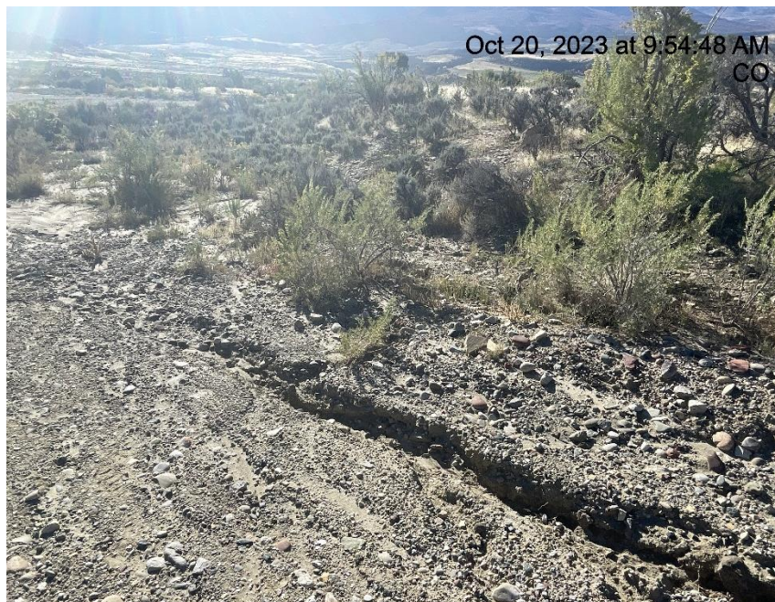
Photo # 3458 Erosion & transport of sediment off lease road into a vegetated area choking off vegetation/insufficient BMP's
