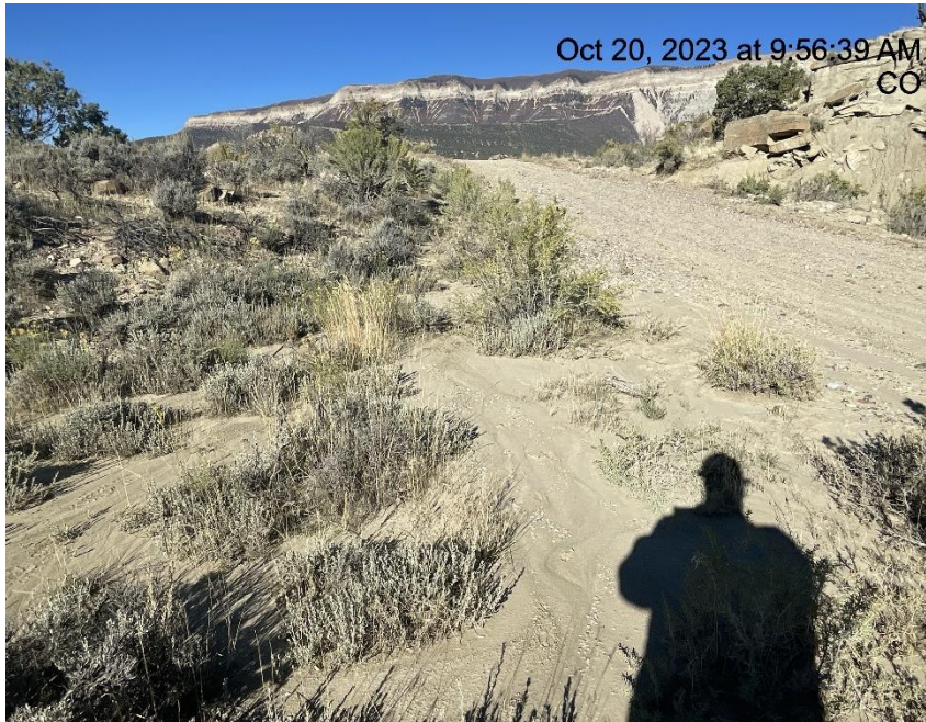
Photo # 3466 Erosion & transport of sediment off lease road into a vegetated area choking off vegetation/insufficient BMP's
