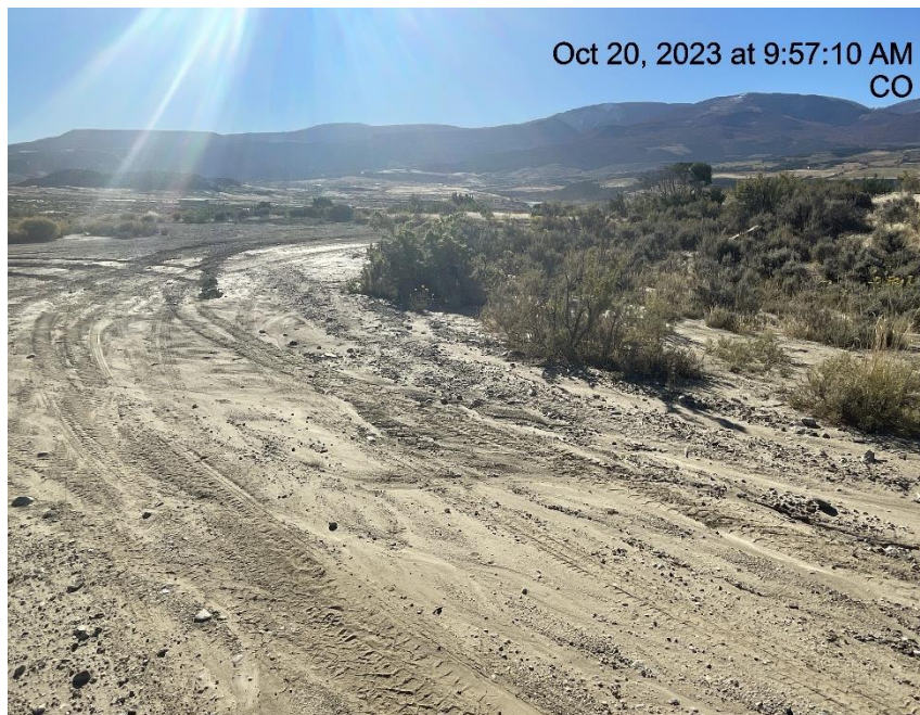
Photo # 3472 Erosion & transport of sediment off lease road into a vegetated area choking off vegetation/insufficient BMP's
