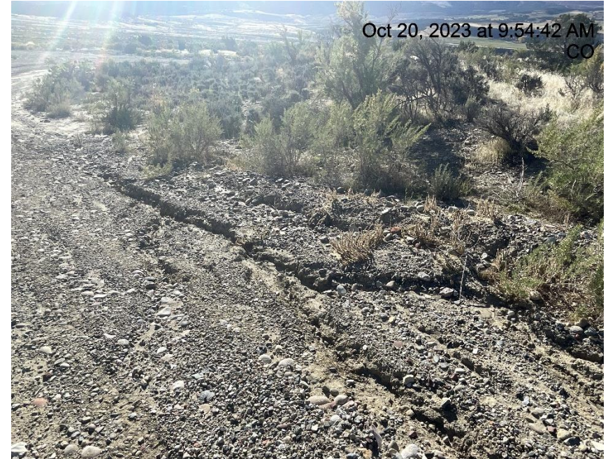
Photo # 3457 Erosion & transport of sediment off lease road into a vegetated area choking off vegetation/insufficient BMP's
