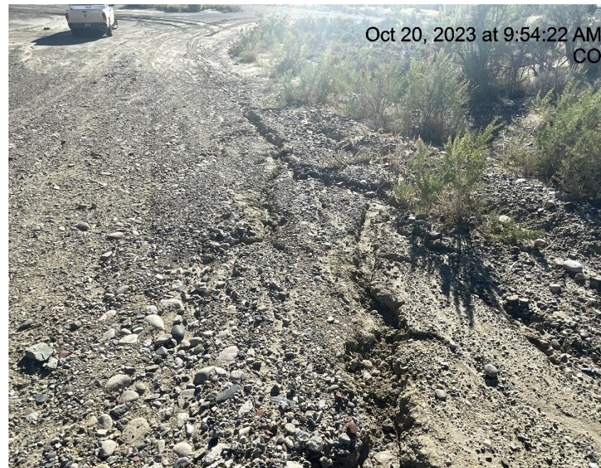
Photo # 3455 Erosion & transport of sediment off lease road into a vegetated area choking off vegetation/insufficient BMP's
