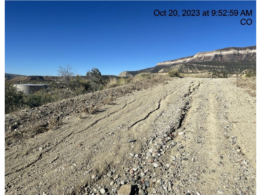
Photo # 3451 Erosion & transport of sediment on lease road /insufficient BMP's
