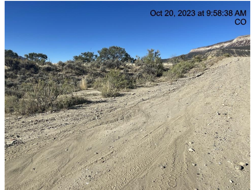
Photo # 3475 Erosion & transport of sediment off lease road into a vegetated area choking off vegetation/insufficient BMP's
