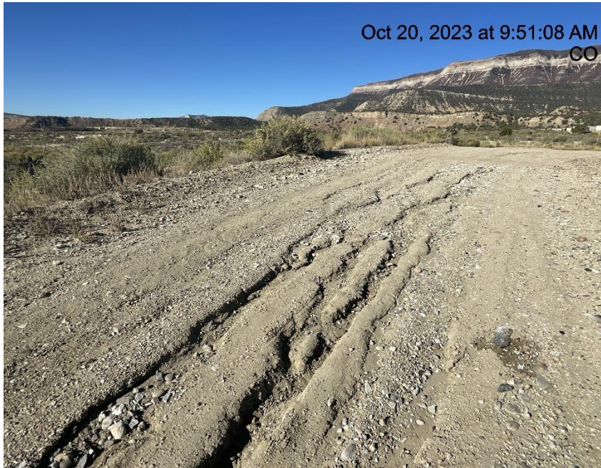
Photo # 3446 Erosion & transport of sediment on lease road /insufficient BMP's
