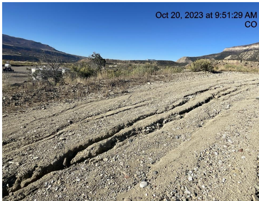
Photo # 3448 Erosion & transport of sediment on lease road /insufficient BMP's
