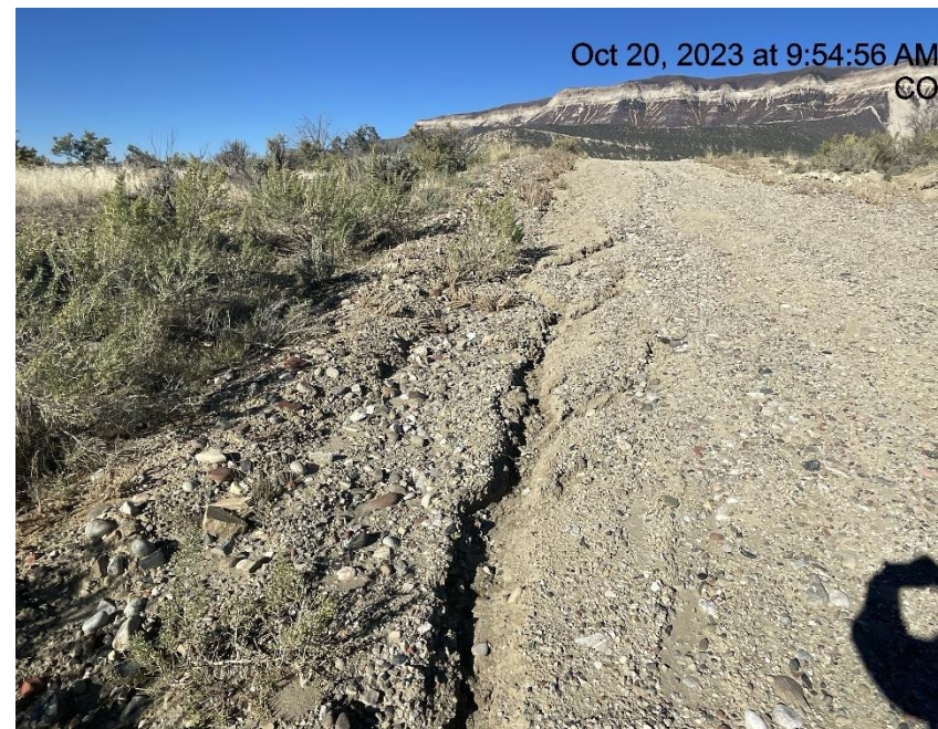
Photo # 3459 Erosion & transport of sediment off lease road into a vegetated area choking off vegetation/insufficient BMP's
