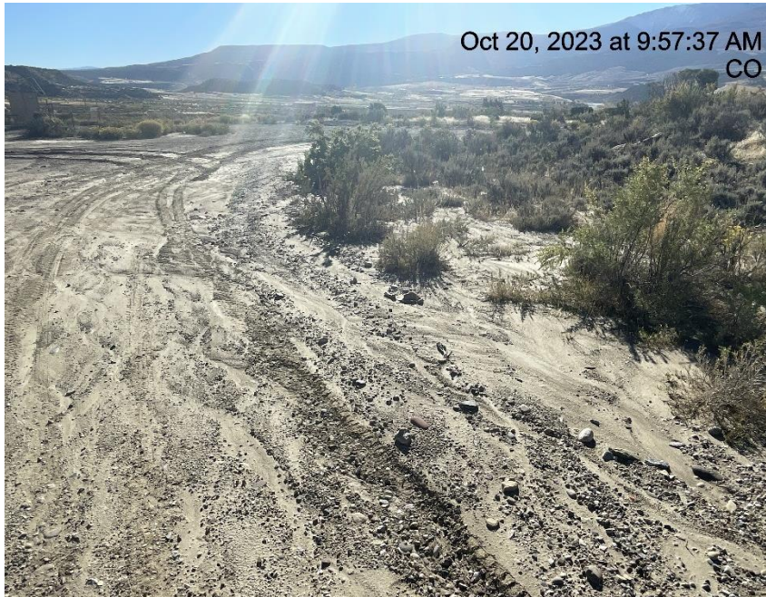
Photo # 3474 Erosion & transport of sediment off lease road into a vegetated area choking off vegetation/insufficient BMP's
