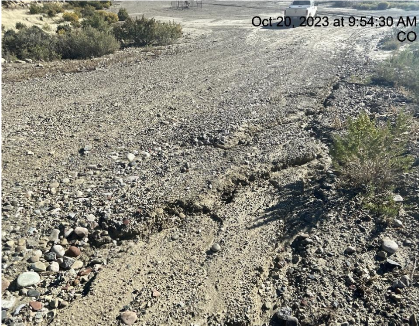
Photo # 3456 Erosion & transport of sediment off lease road into a vegetated area choking off vegetation/insufficient BMP's
