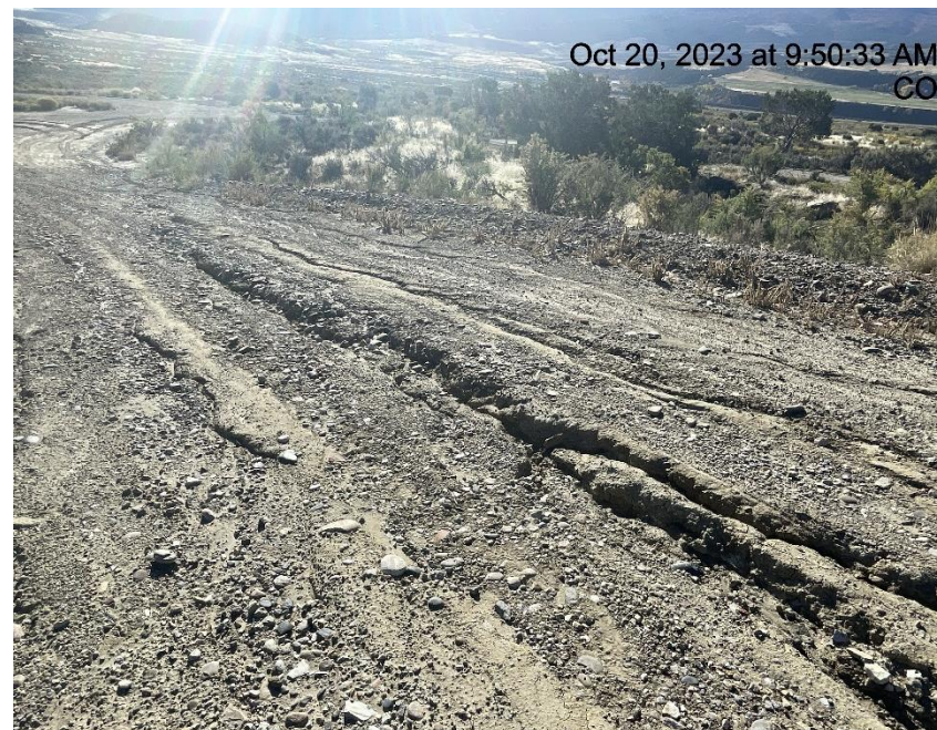
Photo # 3445 Erosion & transport of sediment on lease road /insufficient BMP's
