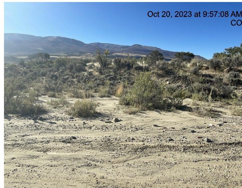
Photo # 3471 Erosion & transport of sediment off lease road into a vegetated area choking off vegetation/insufficient BMP's
