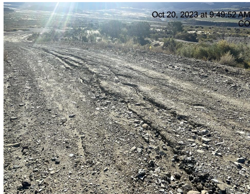
Photo # 3441 Erosion & transport of sediment on lease road /insufficient BMP's
