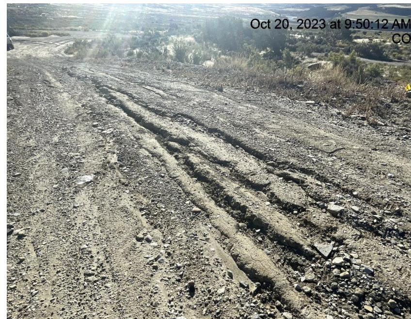
Photo # 3443 Erosion & transport of sediment off lease road into a vegetated area choking off vegetation/insufficient BMP's
