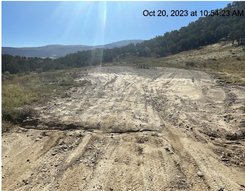
Photo # 3590 Ditch needs maintenance (runs across entrance to location)
