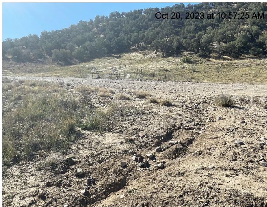
Photo # 3596 Erosion & transport of sediment off location
