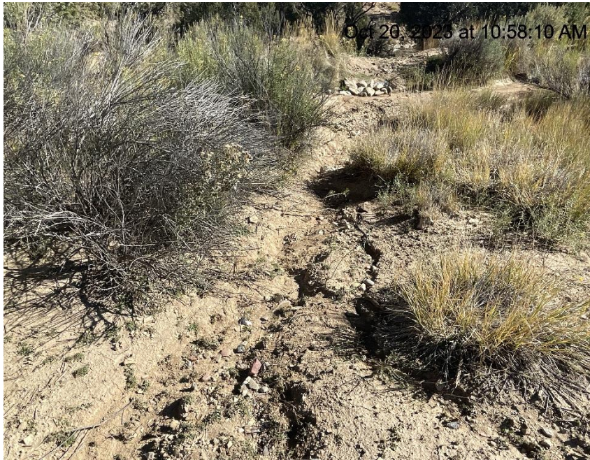
Photo # 3598 Erosion & transport of sediment off location into the interim area choking off vegetation & erosion in the interim area
