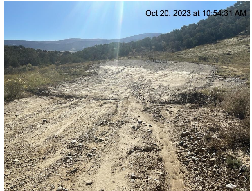
Photo # 3591 Ditch needs maintenance (runs across entrance to location)
