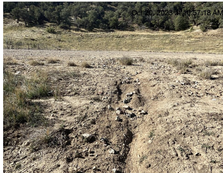
Photo # 3595 Erosion & transport of sediment off location
