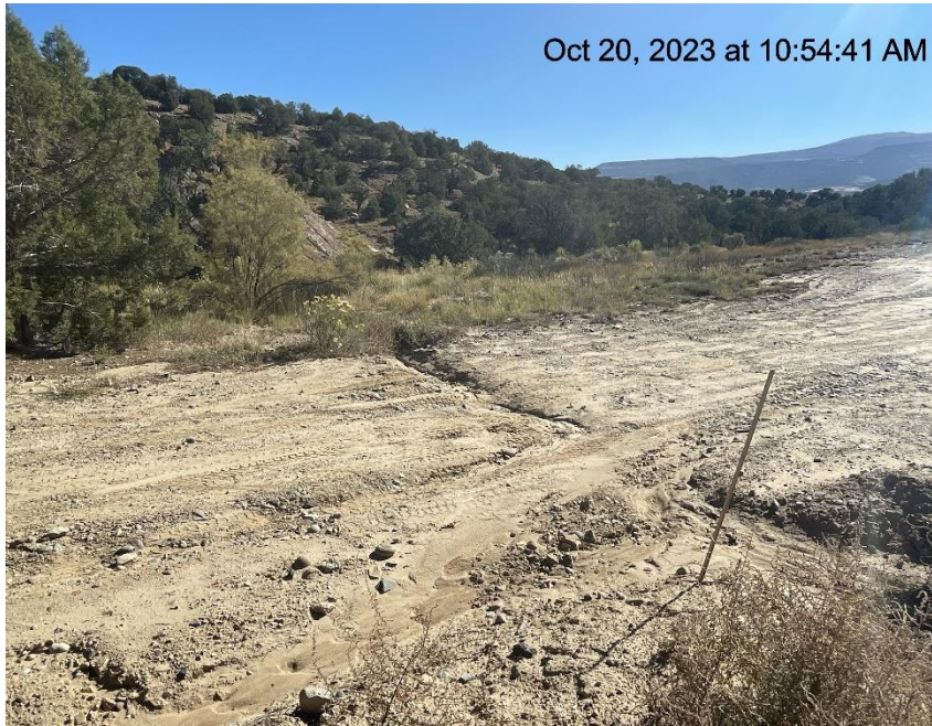
Photo # 3592 Ditch needs maintenance (runs across entrance to location)
