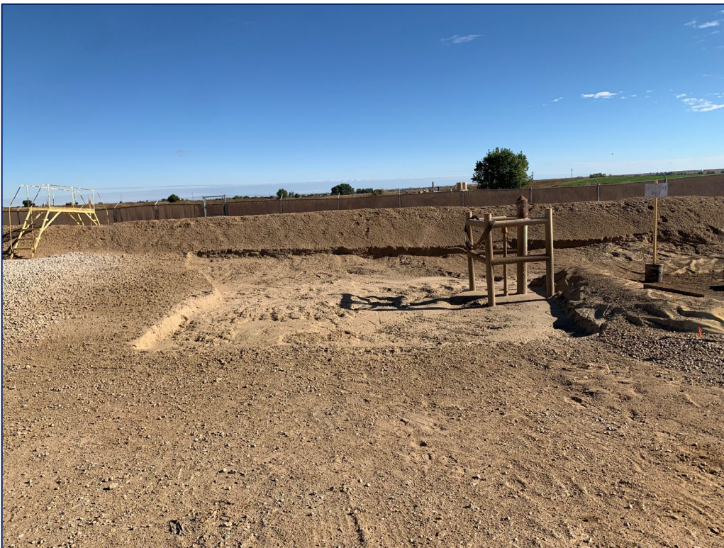
Photograph 2: Area of hydrovaced soil removal. South of northwest corner facing northeast.
