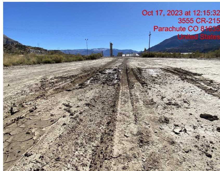
Lack of Stabilization – Photo #07041
