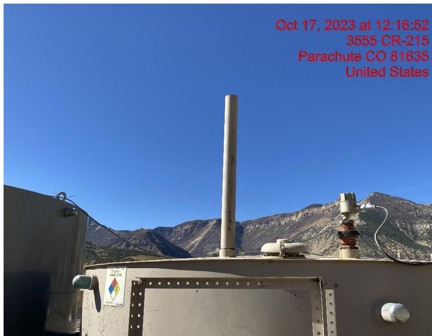
Open-Ended Vent Line – Photo #07044
