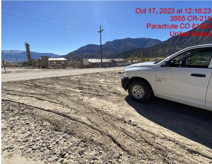
Insufficient Vehicle Tracking BMPs at Location Entrance/Exit – Photo #07050
