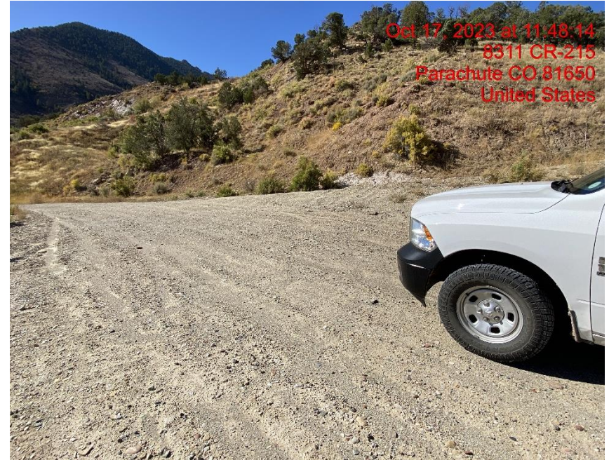
Insufficient Vehicle Tracking BMPs at Location Entrance/Exit – Photo #07019
