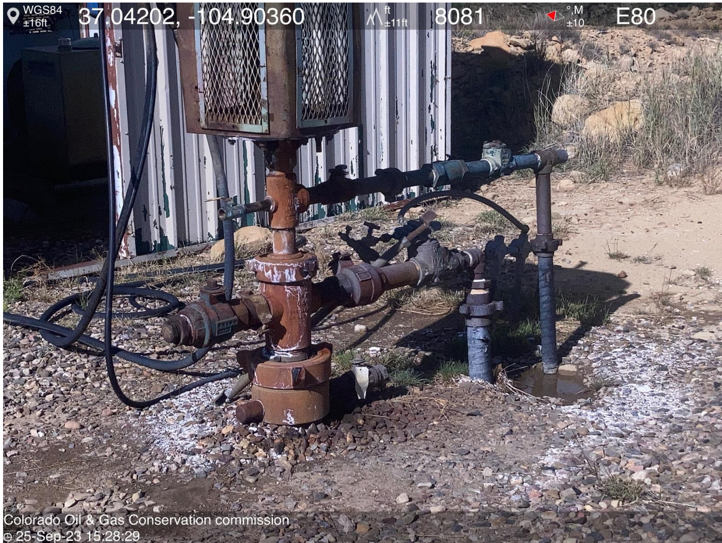
PHOTO 4: Signs of recent slow leak from wellhead. Salt/mineral buildup is evident on the wellhead and ground around wellhead. Securely fasten all valves, pipes, fittings, and Production Facilities to ensure good mechanical condition, inspect at regular intervals, remove salt/mineral buildup, maintain in good mechanical condition remove and dispose of impacted material per Rule 608.e. ca date 11-20-2-23.
