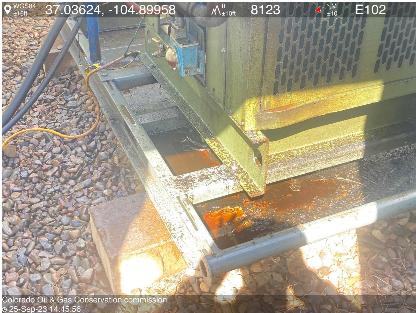
PHOTO 6: OILY WASTE IN ENGINE SKID. COMPLY WITH RULE 1002.f.(2)B, Comply with general provisions of the oil and gas act for wildlife protection AND SB-181. CA DATE 10-21-2023.
