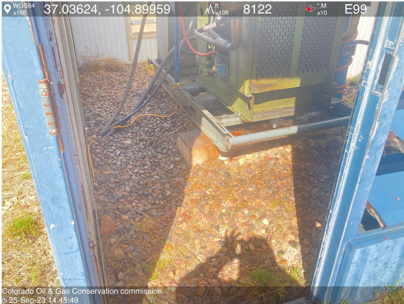
PHOTO 5: AREA OF IMPACTED SOIL NEAR R WELL PRIME MOVER. Conduct maintenance on equipment, cleanup stained material and review self inspection processes. COMPLY WITH RULE 1002,(2).D. CA DATE 11-20-2023.
