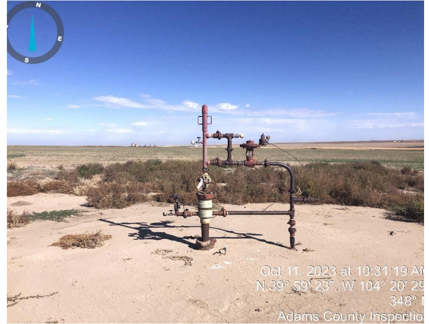
Photo #8 Well head (no sign).
