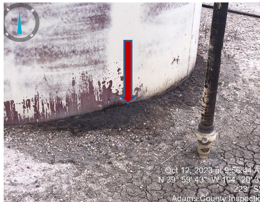
Photo #14 Stained soil under Crude tank.
