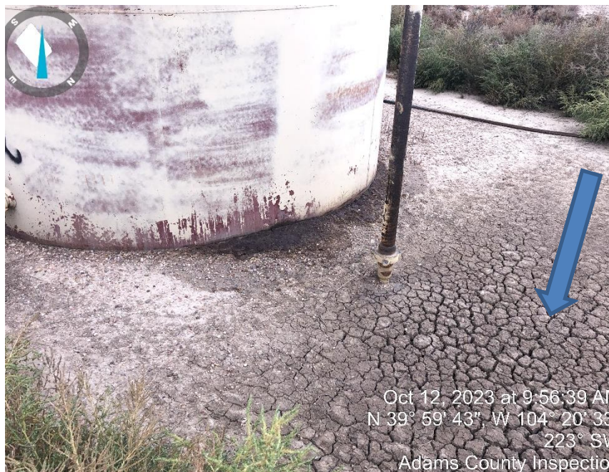
Photo #13 stained soil in berm around crude tanks.
